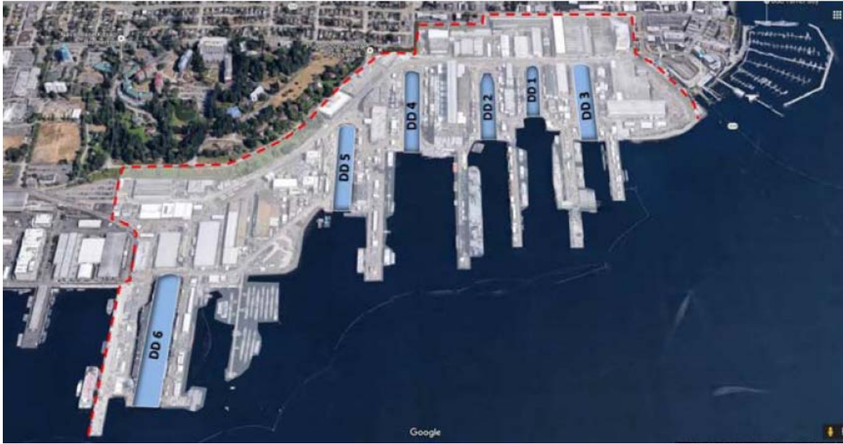
Figure 24: Locations of the six service dry docks at Naval Base (NAVBASE) Bremerton on the Kitsap Peninsula in central Puget Sound.
