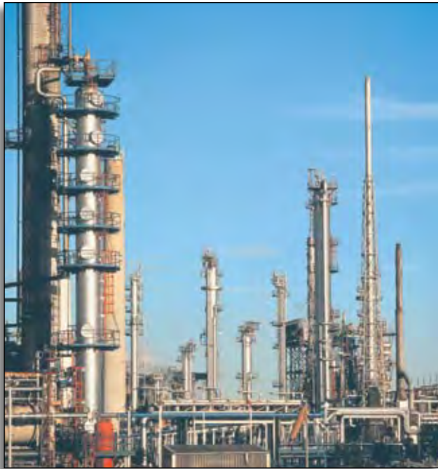
Today's modern refineries and manufacturing complexes often contain both flammable gases and ignitable dusts, making area classification of Division 1 and Division 2 locations an important but tricky task.
