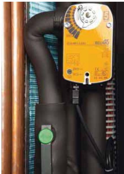
Switchover between a 2 and 3-way valve
