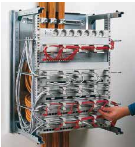
4. Install cables and components
