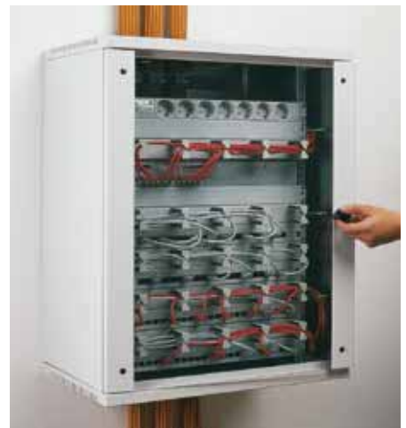
6. Installation is now complete.
