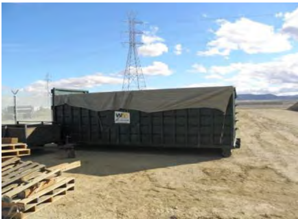
Figure 13: Large properly covered dumpster
