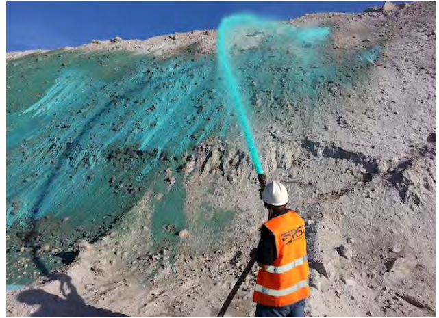
Figure 2. Soil binder and mulch application prior to rain
