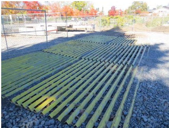
Stabilized Entrance to Staging Area
