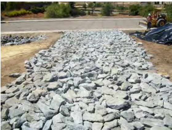
Figure 7: Effective large angular material
