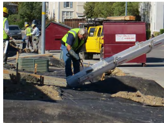
Concrete placement
