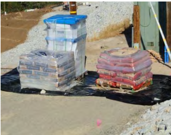
Figure 5: Properly wrapped in plastic, on pallet, and on plastic
