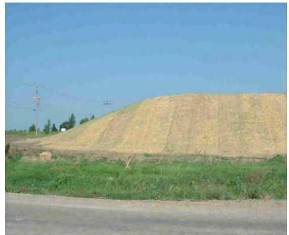
Figure 4. Stockpile stabilized with erosion control blanket
