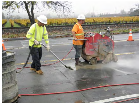
Sawcutting in preparation of excavation
