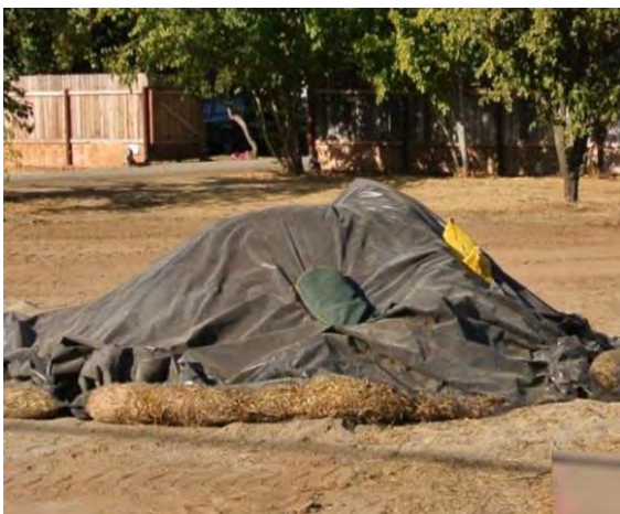
Figure 5. Contaminated stockpile under cover
