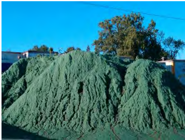
Figure 3. Stockpile stabilized with soil binder and temporary hydraulic mulch
