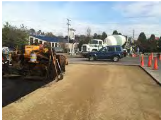
Active Asphalt Paving
