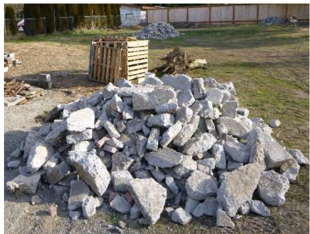
Figure 6. Concrete rubble stockpile in need of cover
