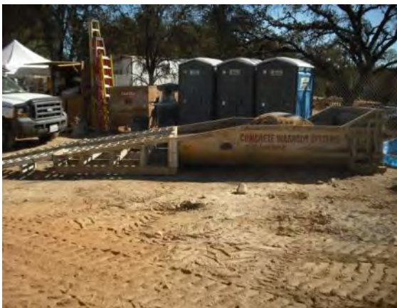
Figure 9: Commercially available washout
