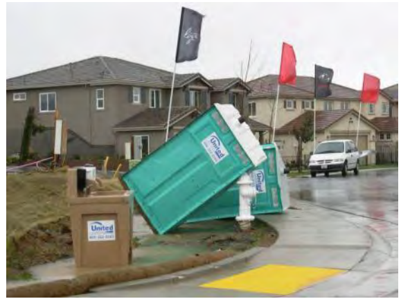
Figure 12: Poor location and protection
