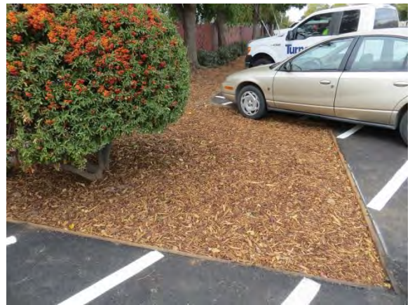
Stabilized disturbed soil area
