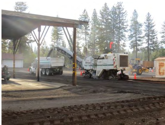
Grinding of existing asphalt
