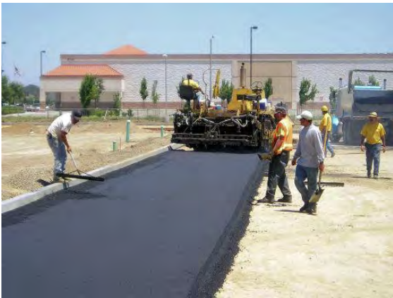
Active Asphalt Paving
