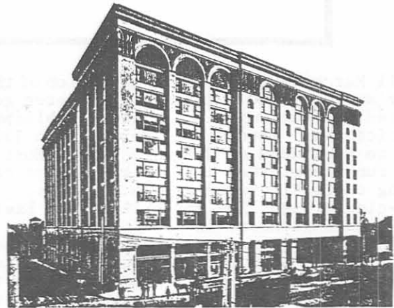
PACIFIC ELECTRIC BUILDING, LOS ANGELES, CALIFORNIA
