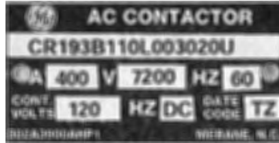
Figure 1. High-Voltage Contactor Nameplate
