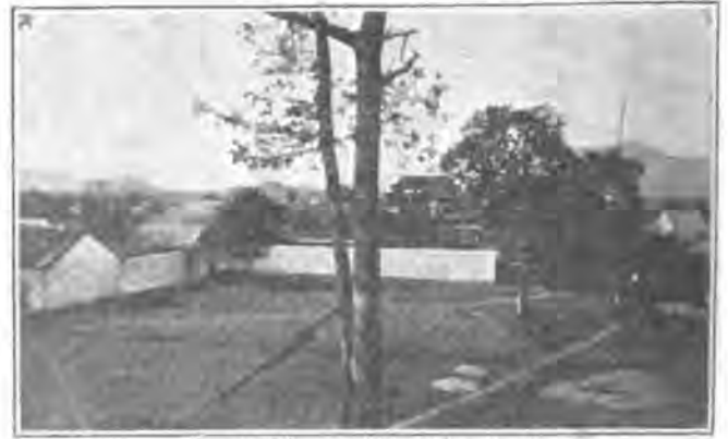
Construction on Shiu Hing Station
