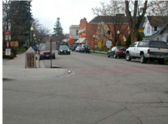
Exhibit 3 - Curb Extension, Boise, ID
