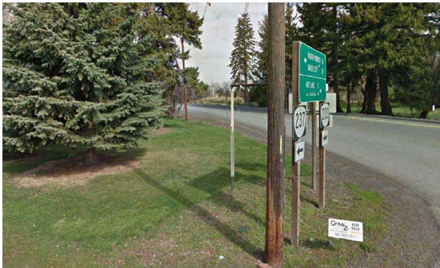
Exhibit 2A Limited Intersection Sight Distance at the OR 203/Bryan Street Intersection; from Bryan Street EB viewing north (top)
