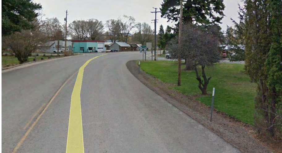
Exhibit 2B Limited Intersection Sight Distance at the OR 203/Bryan Street Intersection; from Bryan Street EB viewing north (top); from OR 203 SB (bottom)
