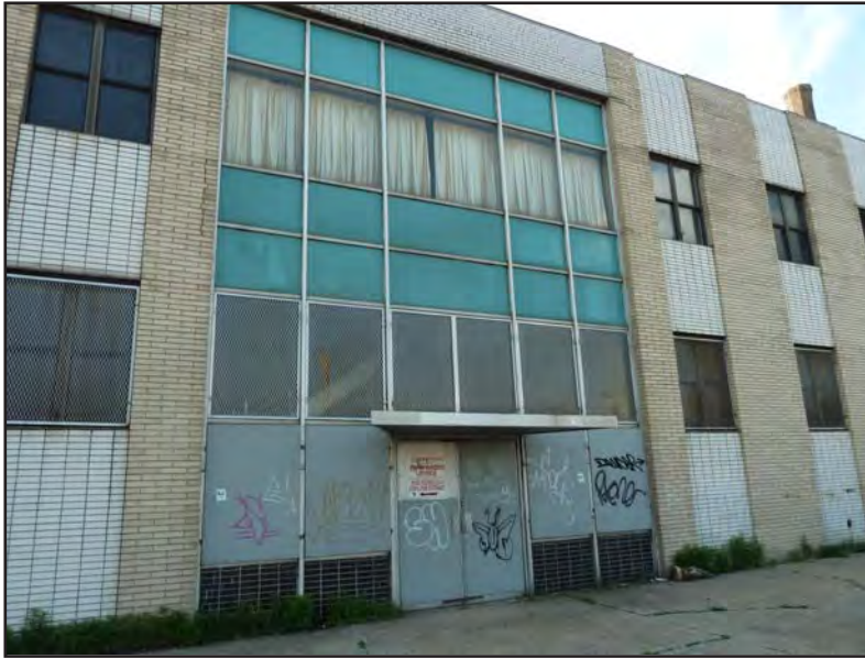
1. Entrance to the existing development site building on Commercial Street.
