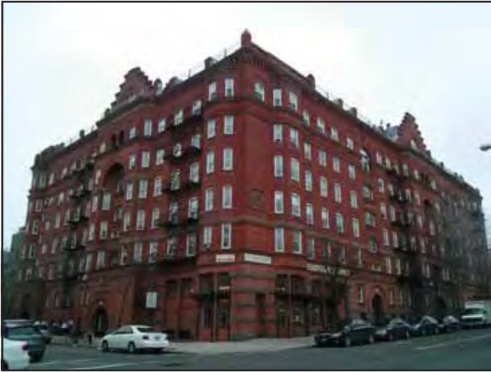
1. The Astral Apartments (view southeast from the intersection of Franklin and India Streets).
