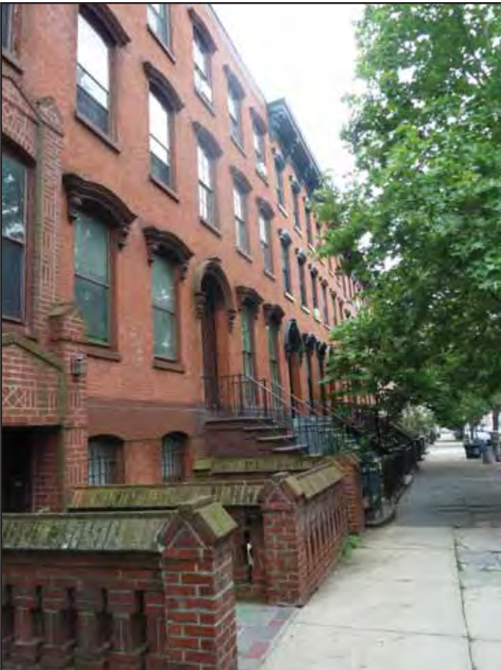
3. 114-124 Kent Street in the Greenpoint Historic District (view west along Kent Street).
