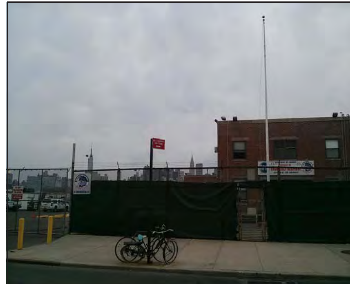
4. View north of the existing NYCTA office building on the City-owned property.
