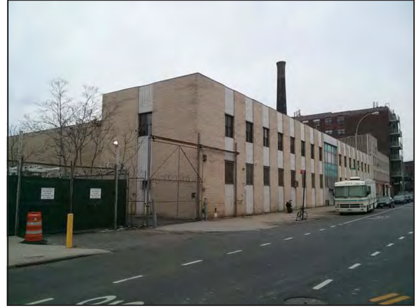
2. View northeast of the development site from Commercial Street.
