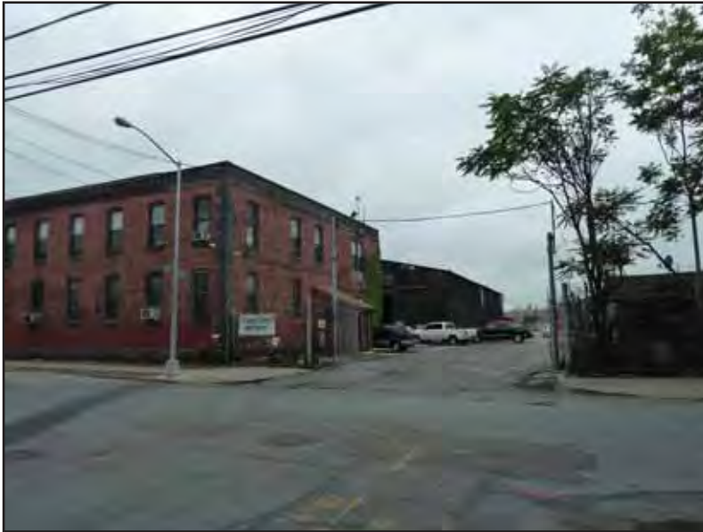
1. View southwest of the intersection of Green and West Streets.
