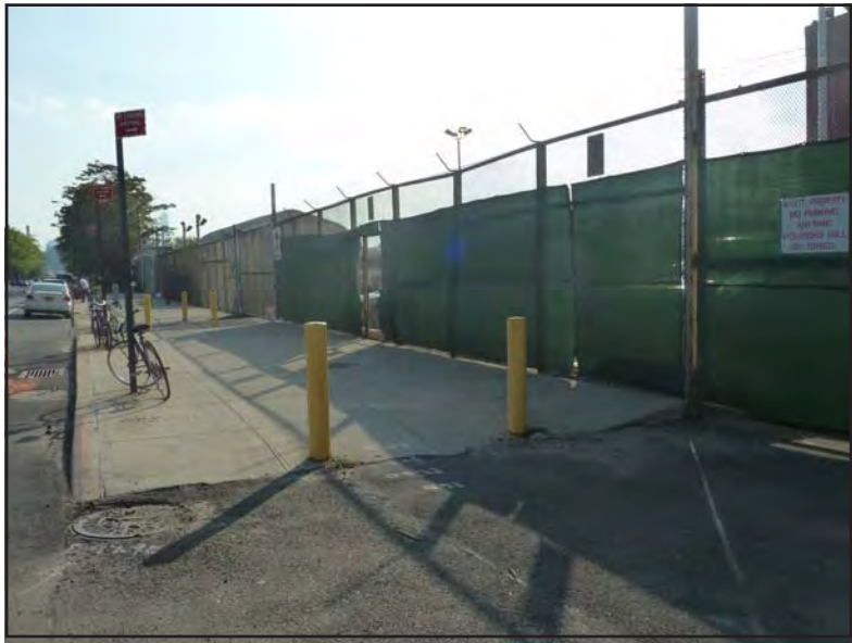
3. View southwest of the sidewalks adjacent to the City-owned property.
