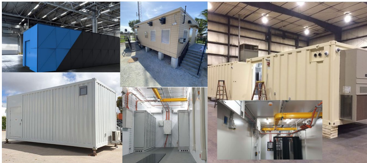
Figure 10-32. Example of a prefabricated power feed equipment shelter.
