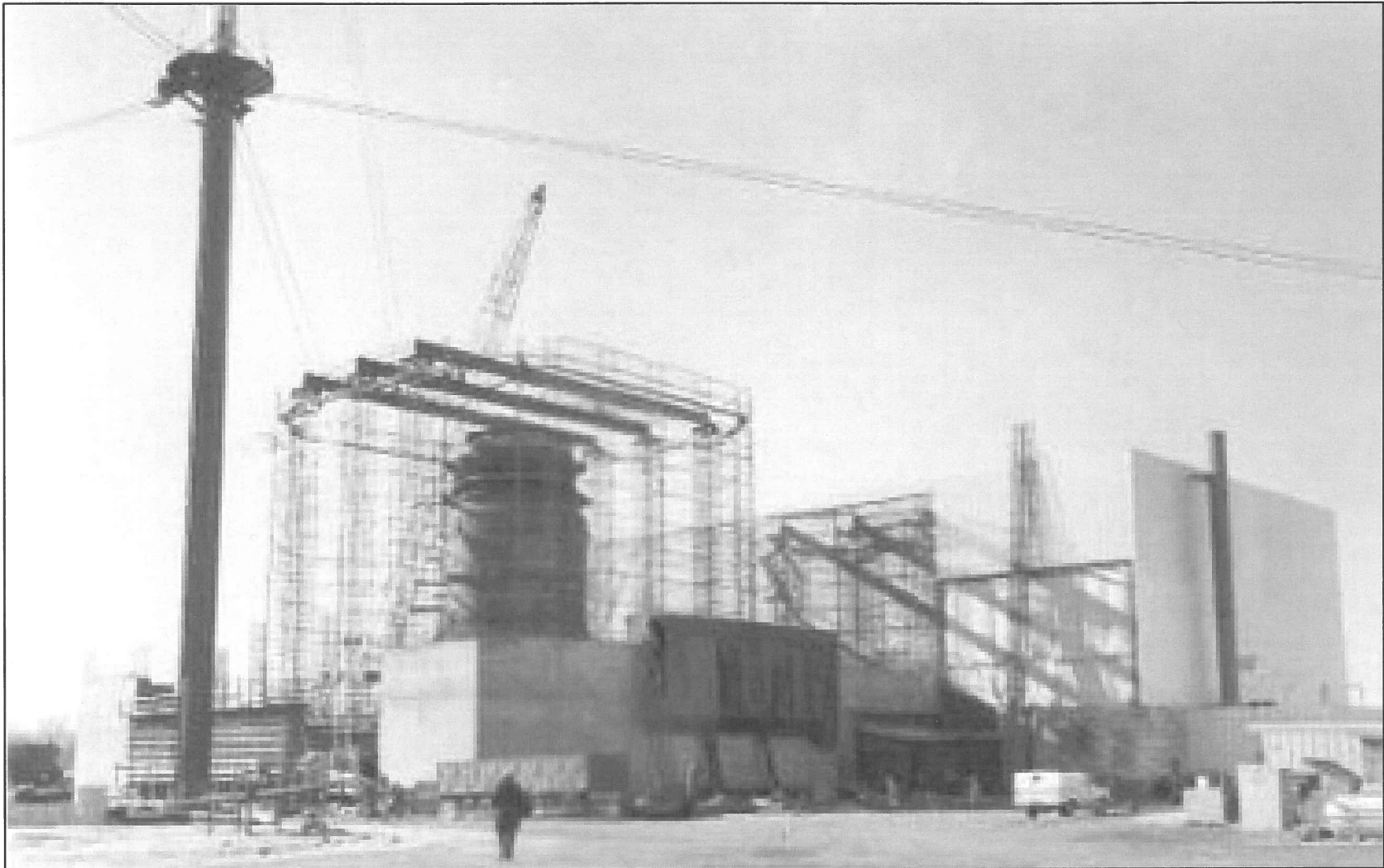
Figure 3.8-6 MNGP Reactor Building Facing West-Northwest, During Construction, 1968
