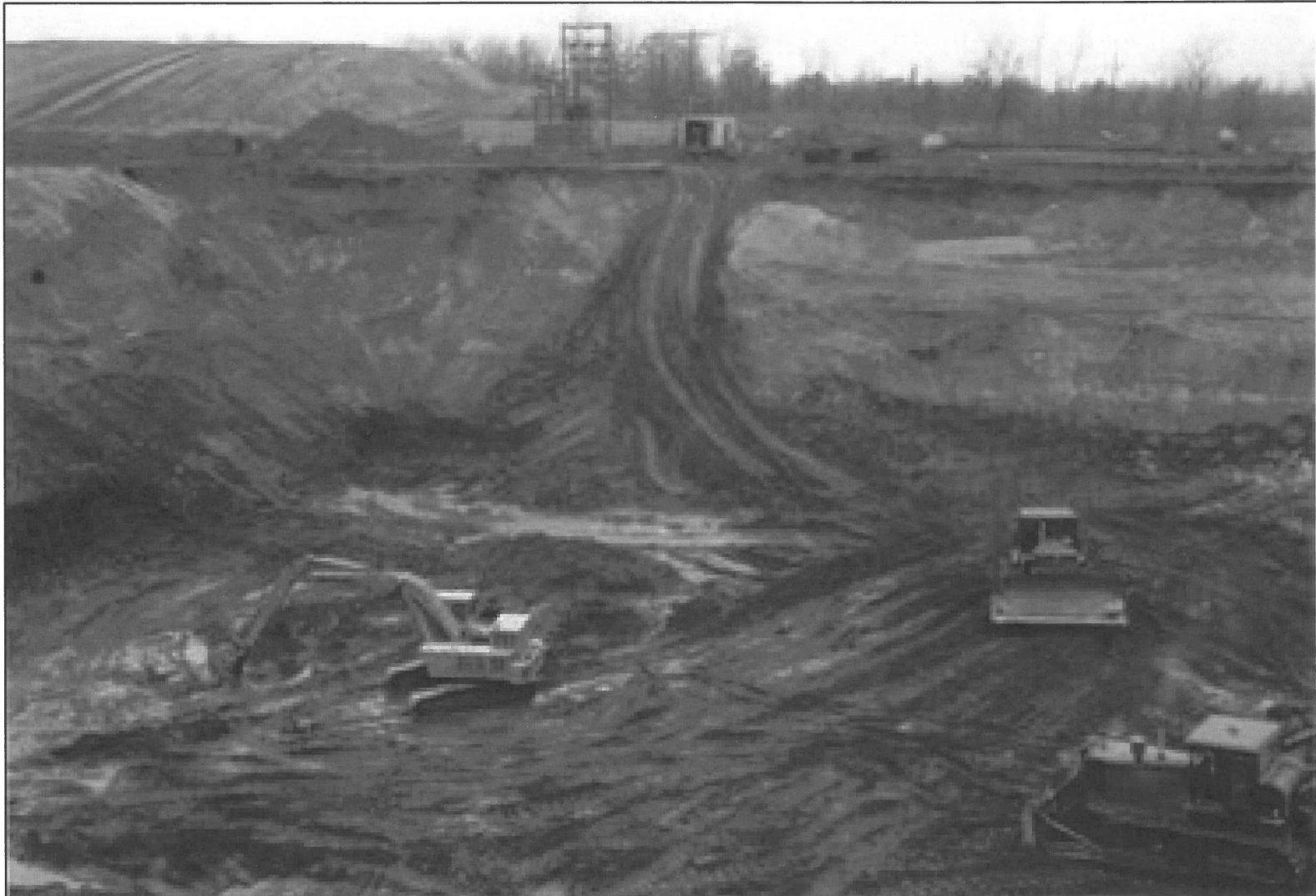
Figure 3.8-5 Facing West-Northwest During Later Phases of Excavation for the Reactor Building, 1966
