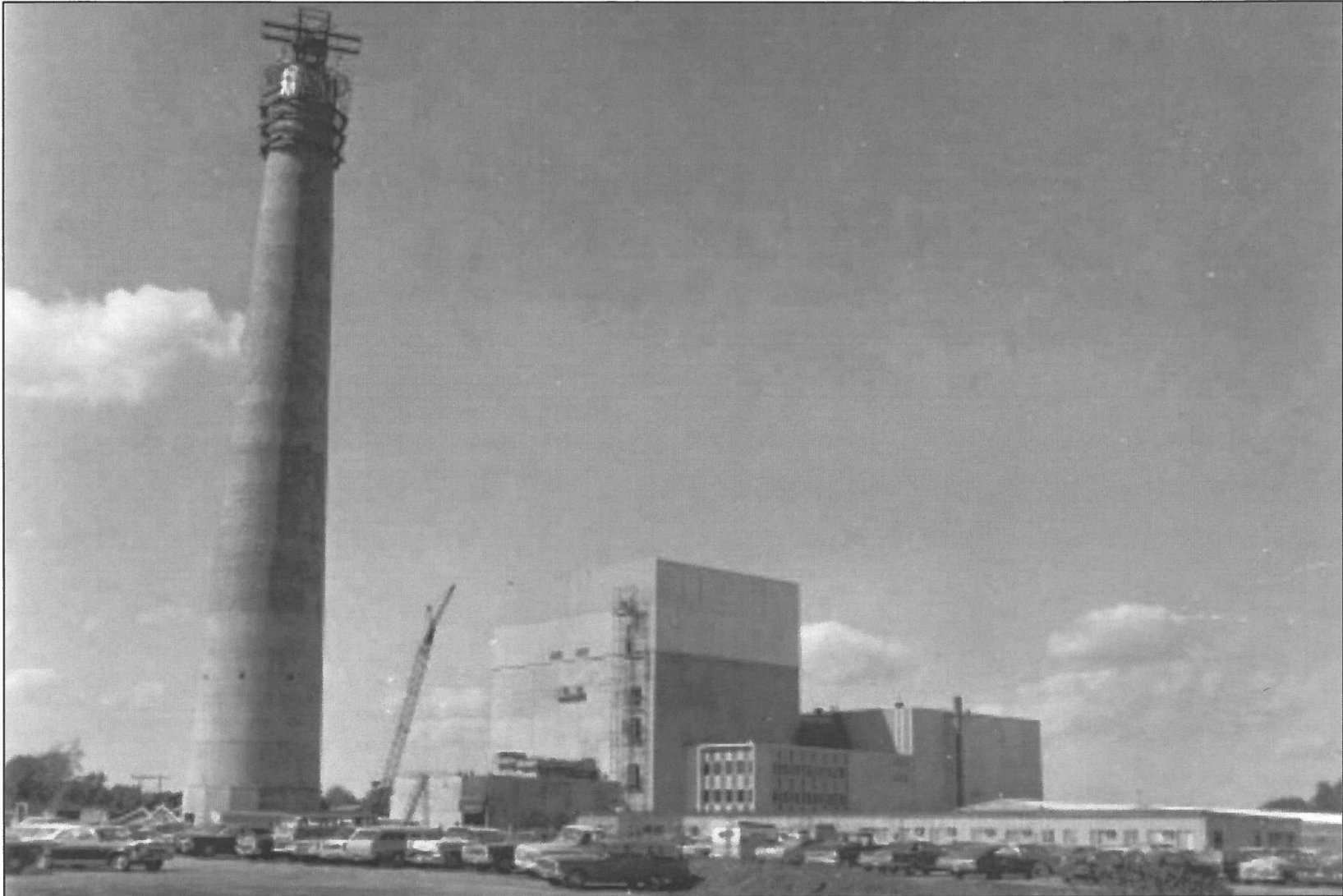
Figure 3.8-7 MNGP Reactor Building Facing West-Northwest near Completion of Construction, 1969
