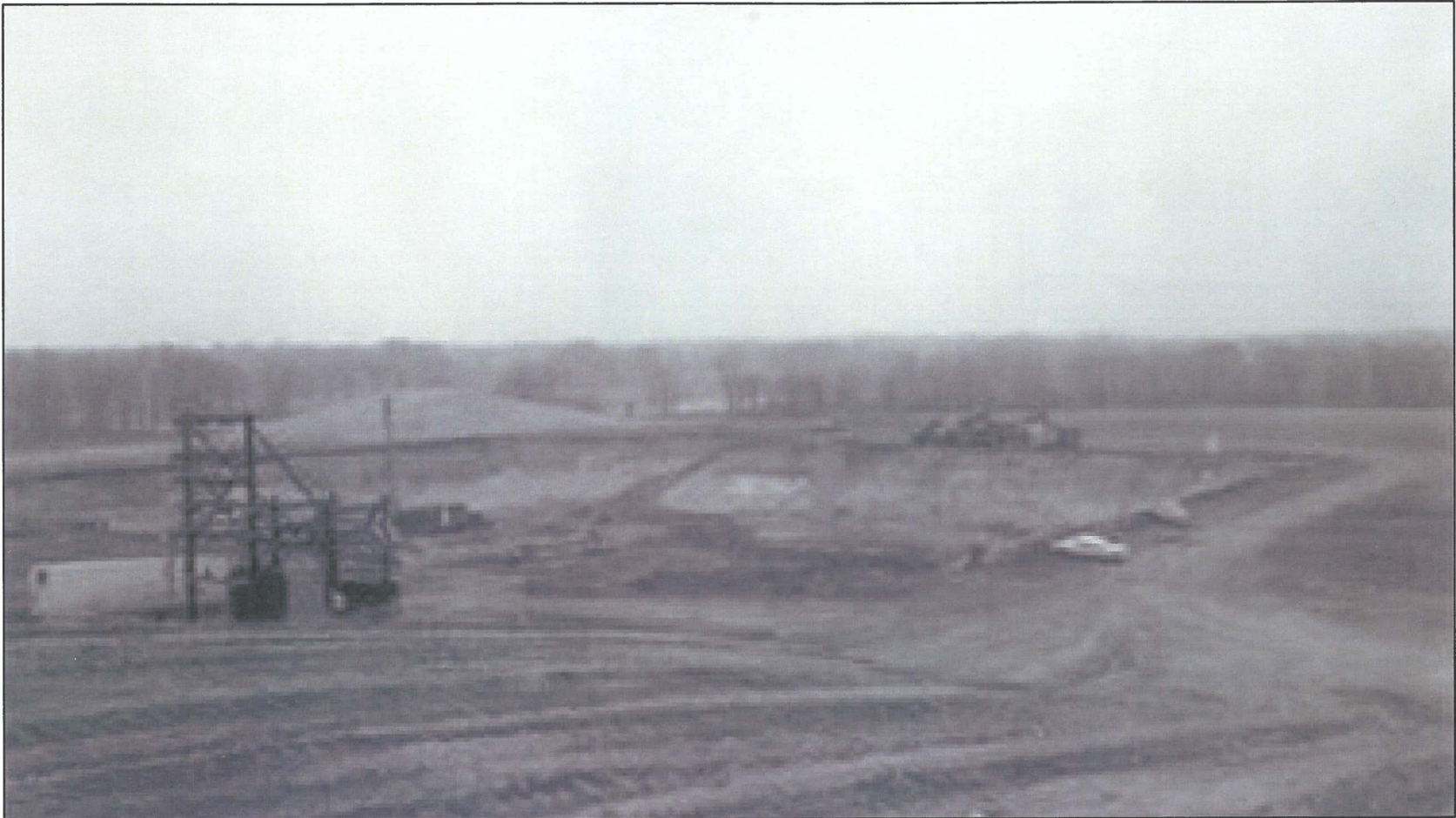
Figure 3.8-4 Facing Northeast During Initial Grading and Excavation at the MNGP Site, 1966
