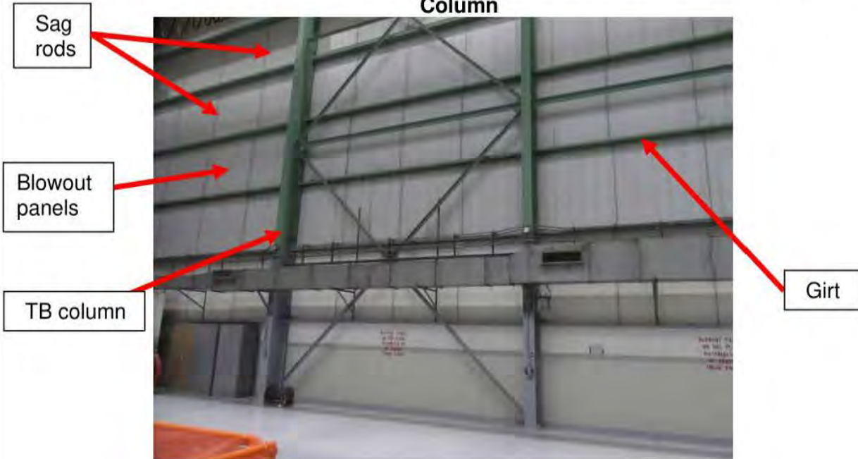
Figure 1-2: General View of the Turbine Building North Wall
