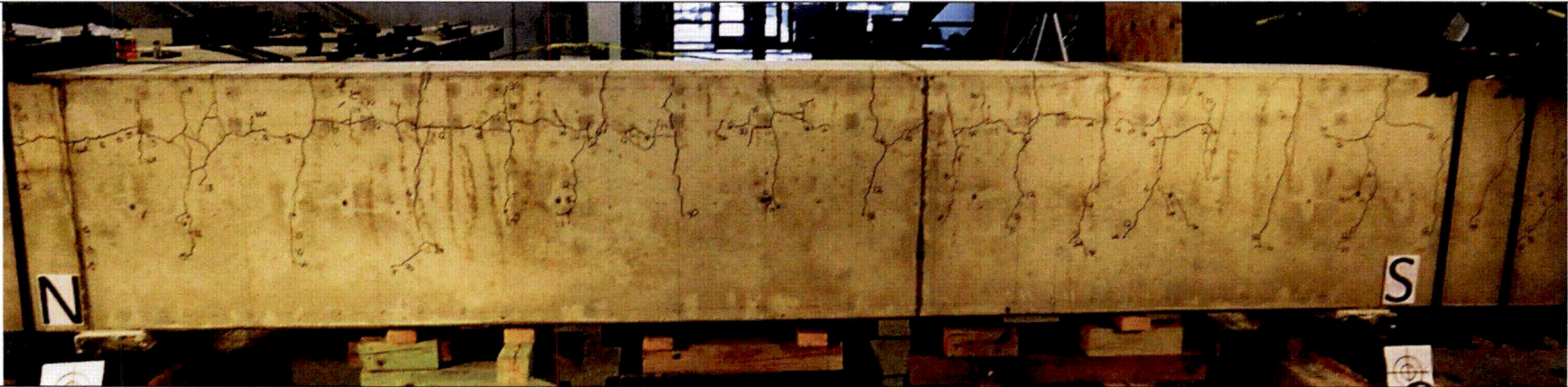
GIRDER B2 – Load = 36 kip.
