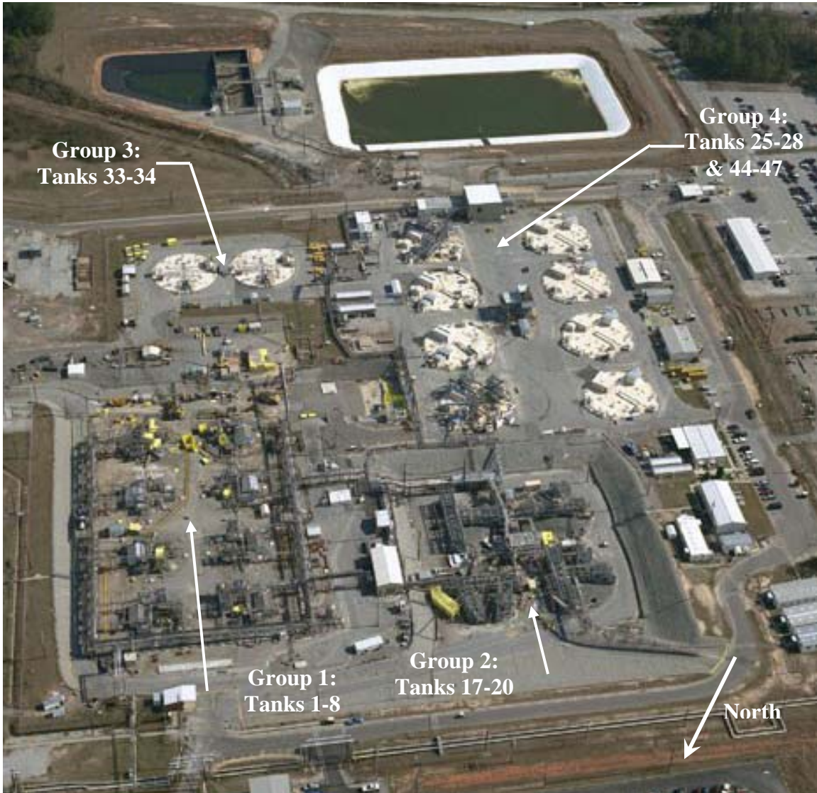
Figure 3. FTF Aerial View
