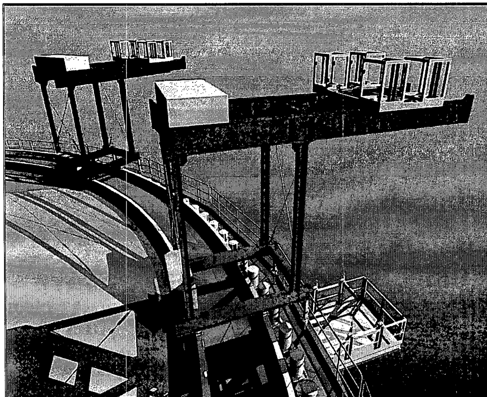
FIGURE 2: UPPER SUPPORT FRAMES INSTALLED ON CONTAINMENT DOME
