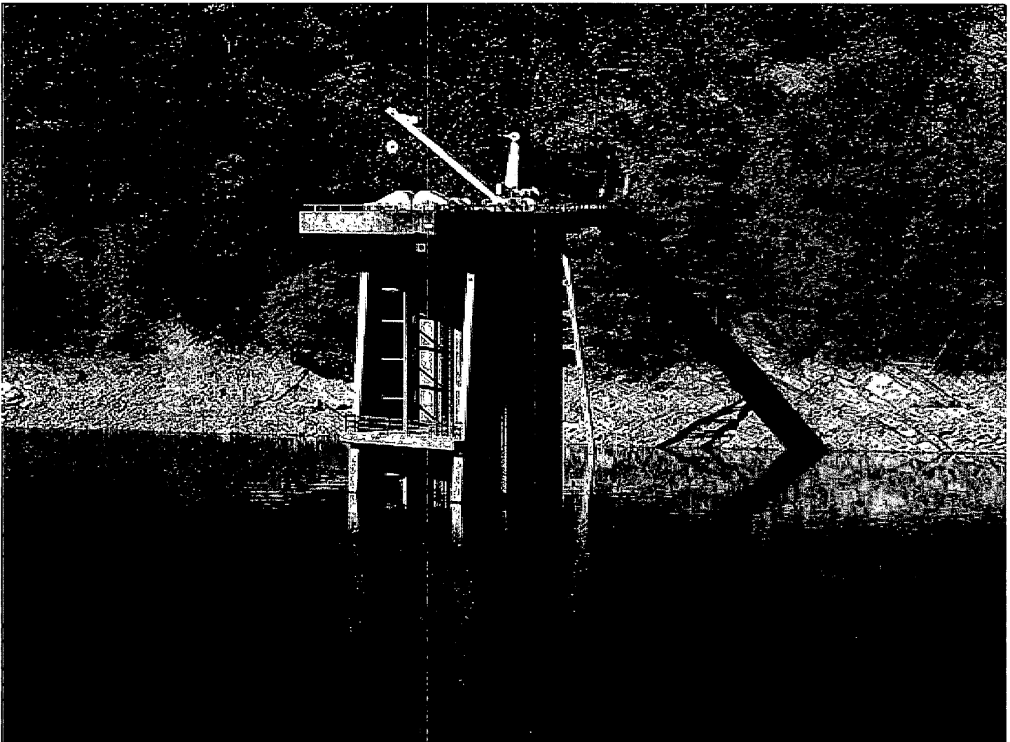
FIGURE 8 - Power Intake Structure near Left Bank, September 1999
