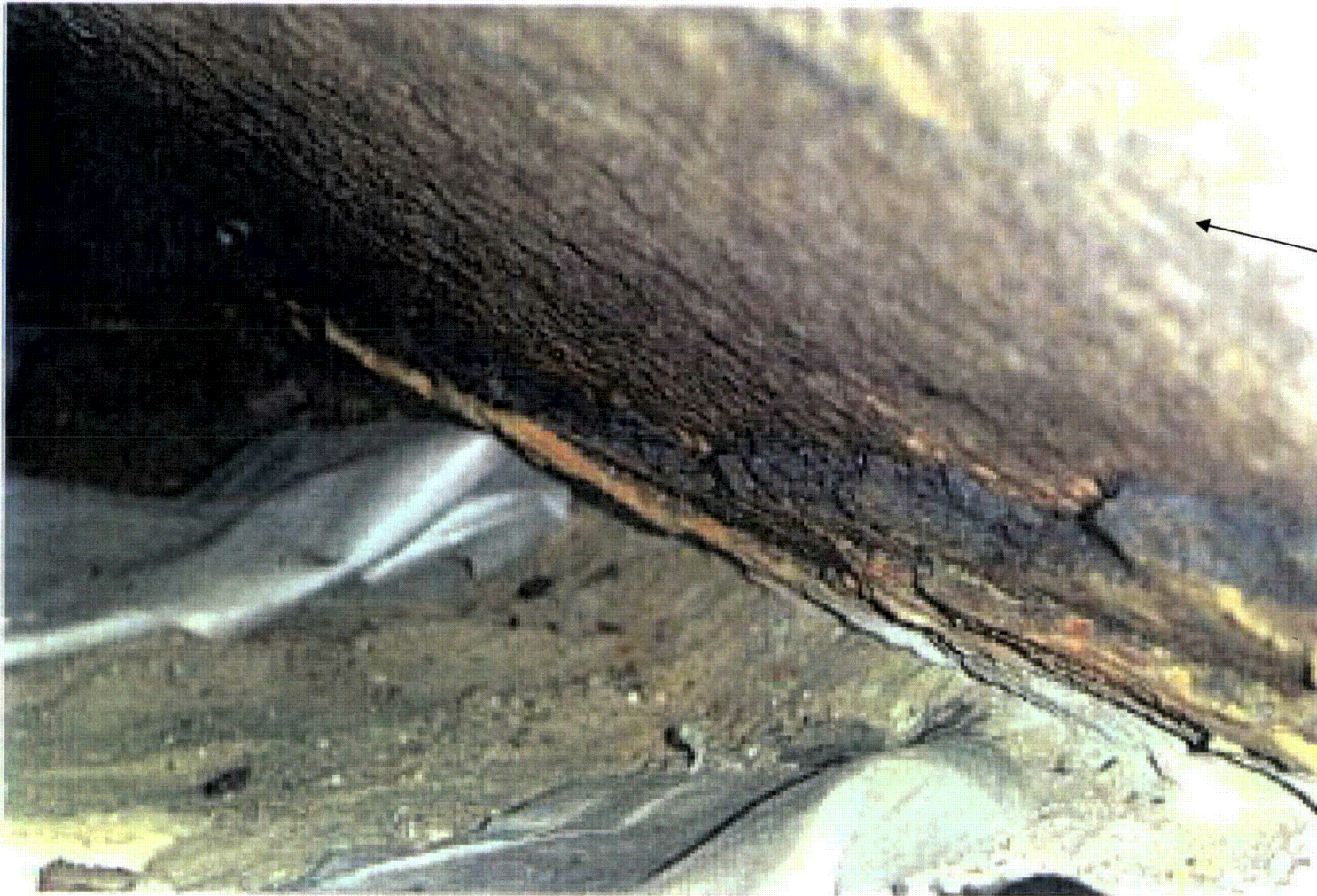
Corrosion product on drywell vessel
