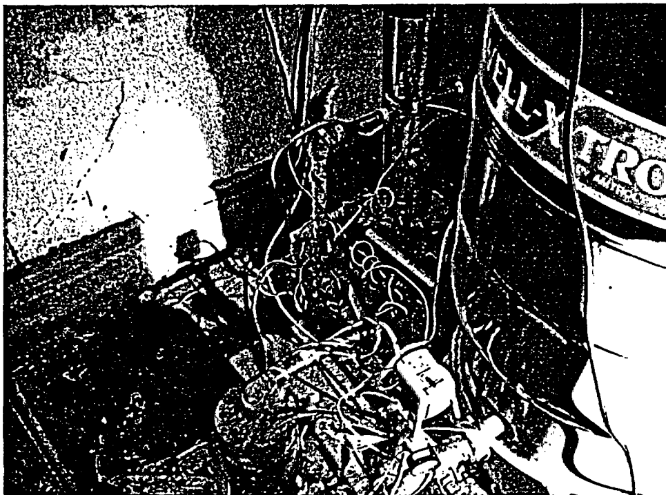
Photographs of a domestic well located at the Clark and Knowles homes on Rendezvous Rd. The DOE identified this well as potentially affected by site contaminants. Well inspection by Northern Arapaho Utilities revealed that this unregulated source was cross-connected into the alternate water supply system.
