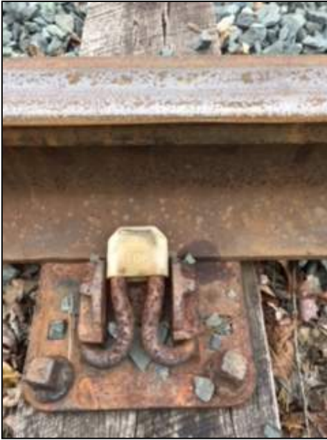
Elastic Fastener: Pandrol Fast Clip
