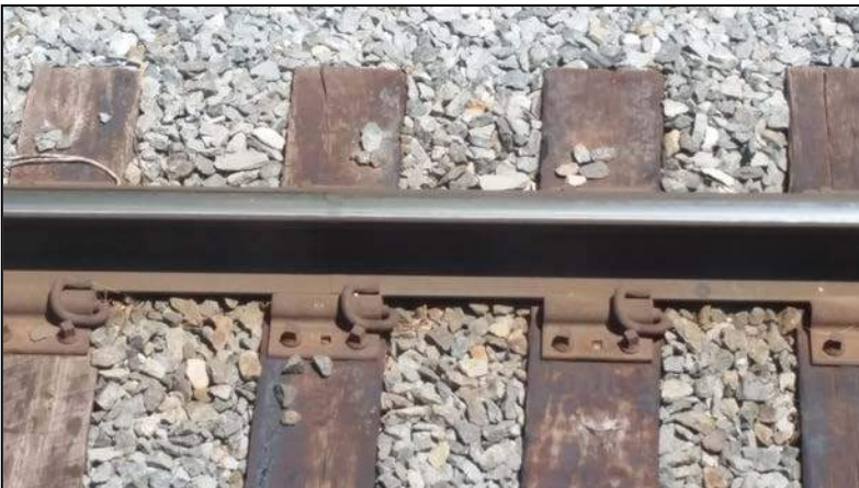
Elastic Fastener: Pandrol E-Clip
