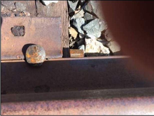
Tie Plate with Anchors Applied Correctly
