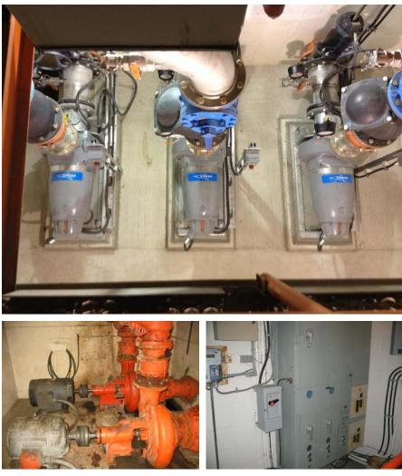
**Top:** The Flygt NZ-3171 pumps installed at Ross Street Station are smaller and sleeker, which makes maintenance easier and safer. **Bottom left:** Parts for the original pumps at Ross Street Station were not readily available, causing long lead times for repairs. **Bottom right:** The project involved completely upgrading mechanical and electrical systems.
