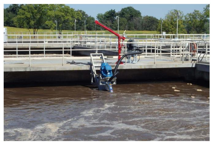
The Universal Mount allows for aerator maintenance to be performed without the need for operators to enter the basin or reach over railing.
