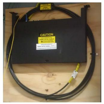
**Above:** Always leave several loops of spare cable in the control panel. **Right:** If a cable is being installed outdoors it will have a stronger jacket/ armouring on it.
