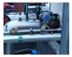
A 454FTB WGF unit was installed to measure output from the acid fermentation tank.
