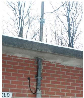
it is more common for the messenger wire to have to be installed separately.
