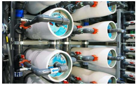
Pre-treatment removes contaminants, which helps the RO membranes resist fouling.
