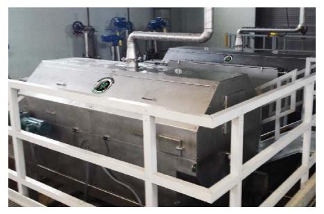
Above: A number of screen designs can be used to protect MBRs, including rotary drum and band screens. **Right:** MBR fouling.
