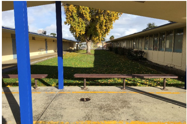
#10 EXTERIOR UNITS 1 AND 2
