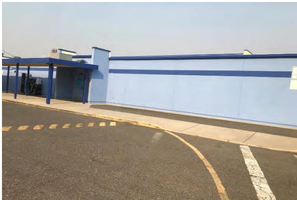
#5 SIDE OF MULTIPURPOSE BUILDING
