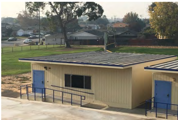
#23 ROOF AT PORTABLES
