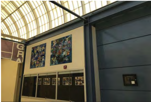
#31 STEEL FRAMING, ARCHED SKYLIGHT, BUILDING 300
