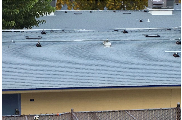
#14 ASPHALT ROOFING
