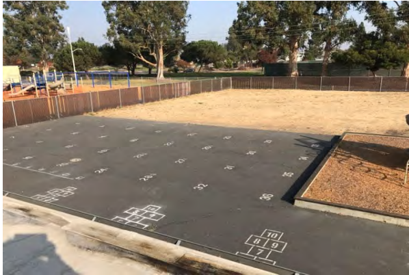
#13 ASPHALT PLAY SURFACE
