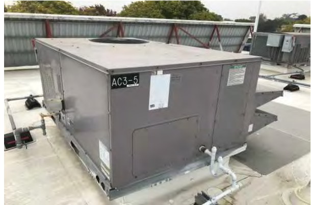
#32 HEAT PUMP, PACKAGED (RTU), 3.5 TO 5 TON
