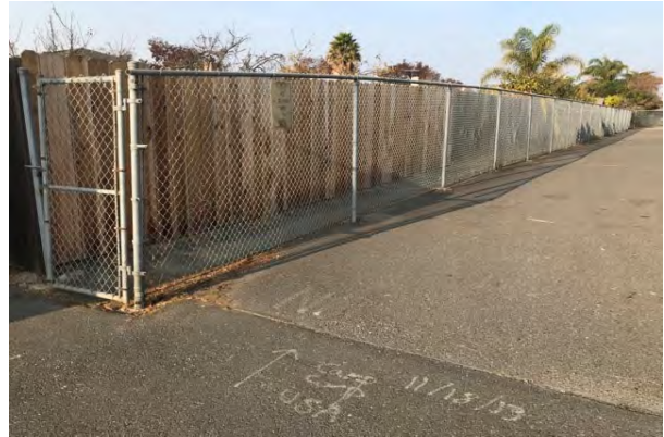
#14 CHAIN LINK FENCE
