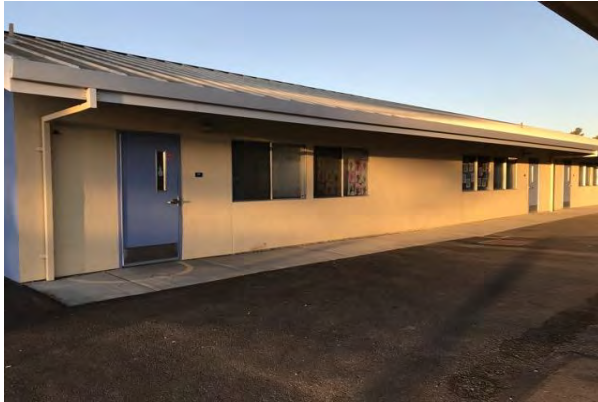
#7 MODULAR CLASSROOM BUILDING
