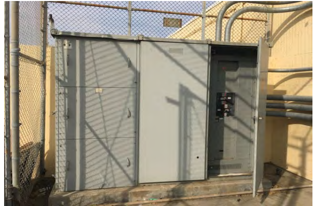
#52 SWITCHGEAR, 2,000 AMP
