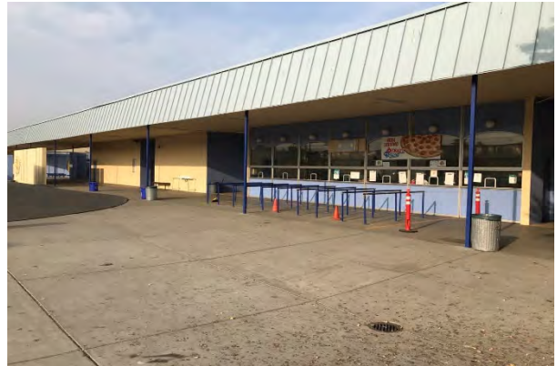
#4 SNACK BAR, GYMNASIUM BUILDING
