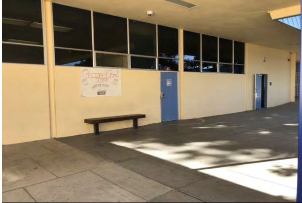
#25 EXTERIOR WALL, PAINTED SURFACE
