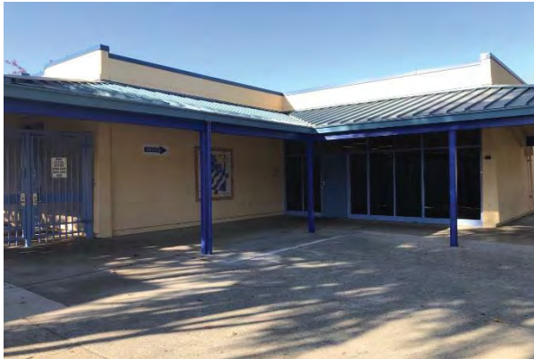
#3 FRONT ENTRY, OFFICE (100)
