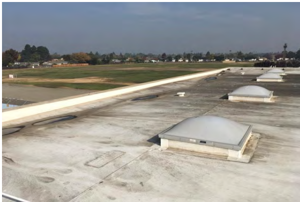
#21 ROOF, SINGLE-PLY TPO/PVC MEMBRANE
