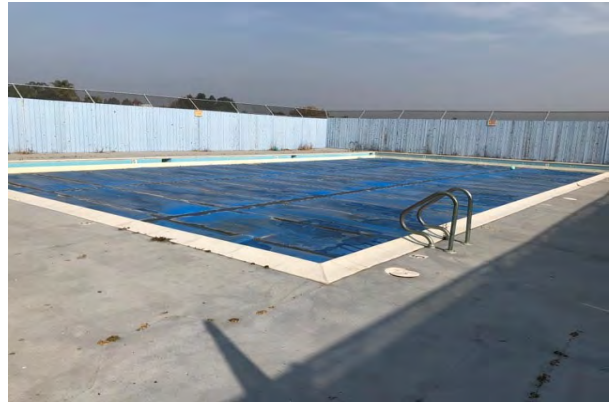
#16 SITE IMPROVEMENTS, POOL ABANDONED IN PLACE
