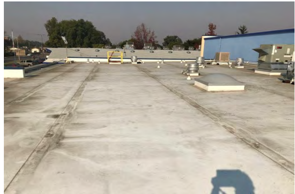
#22 TPO AT MULTIPURPOSE BUILDING
