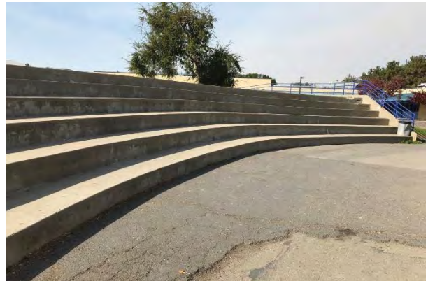
#18 UNEVEN WALKING SURFACES
