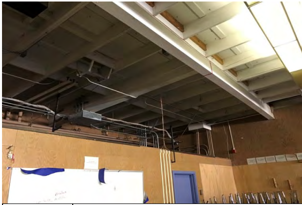
#19 STRUCTURE, WOOD FRAMED ROOF
