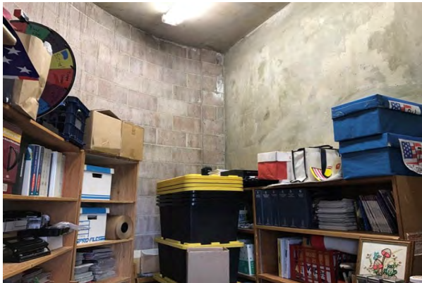
#17 STRUCTURE, CAST CONCRETE AND CONCRETE BLOCK
