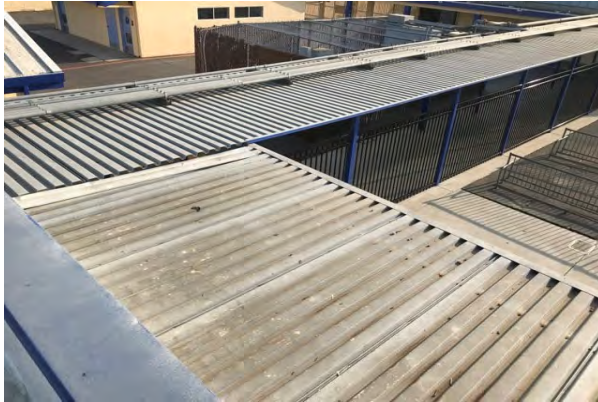
#25 METAL WALKWAY ROOFING
