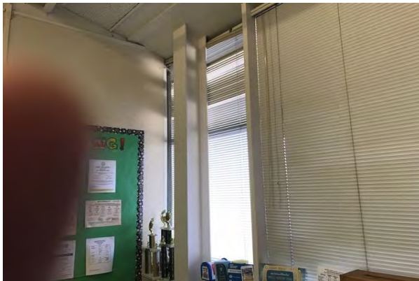
#17 STRUCTURE, STEEL COLUMNS
