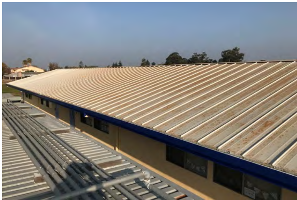
#23 METAL ROOFING AT MODULARS
