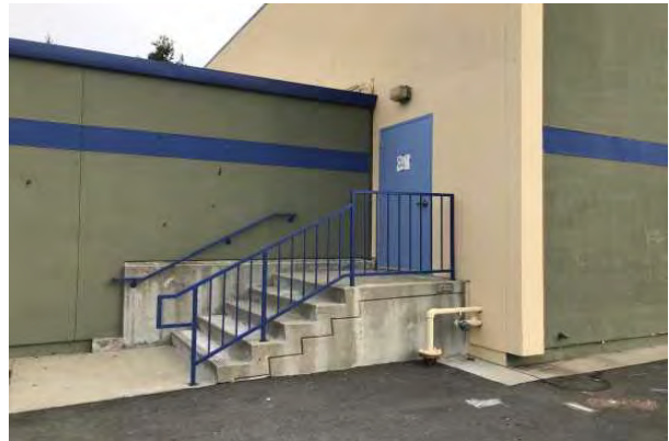
#10 BUILDING 6 - EXTERIOR STAIRS
