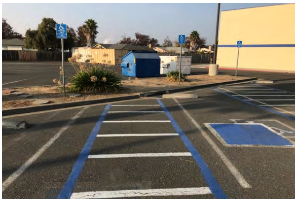
#11 PARKING LOT STRIPING
