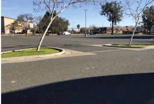
#25 PARKING LOTS, ASPHALT PAVEMENT
