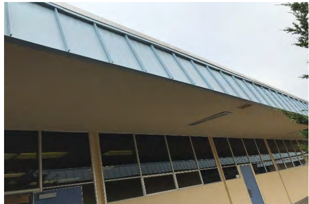
#22 METAL MANSARD ROOF
