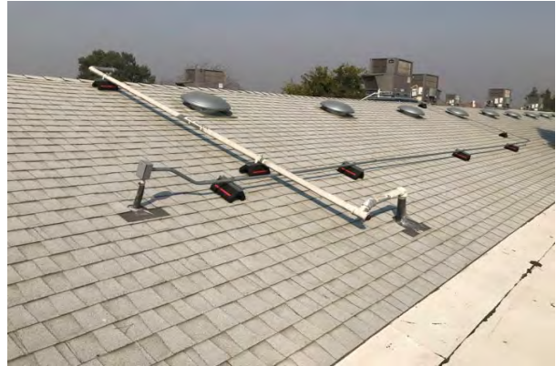
#20 ASPHALT SHINGLES AT BUILDINGS 1, 2 AND 3
