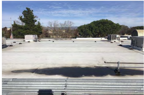
#32 ROOF, SINGLE-PLY TPO
