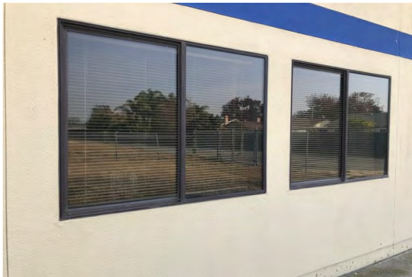
#29 WINDOWS AT MODULARS
