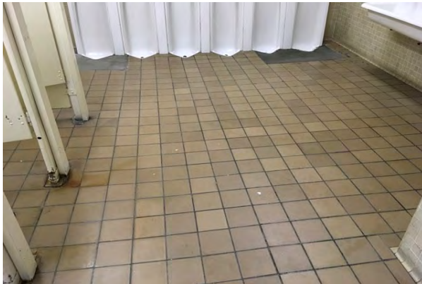
#27 INTERIOR RESTROOM FLOOR FINISH, CERAMIC TILE
