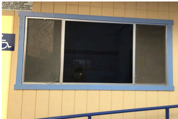
#27 WINDOW AT PORTABLE ALUMINUM DOUBLE-GLAZED
