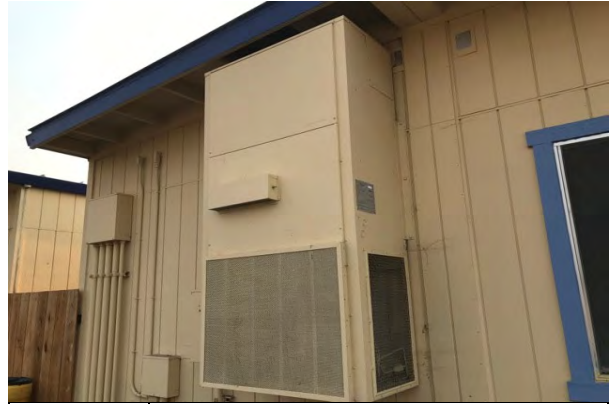
#32 PORTABLES, HEAT PUMP, PACKAGED (RTU)
