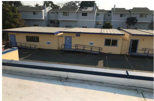
#24 METAL ROOFS AT THE PORTABLES
