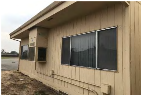
#41 MODULAR - PACKAGED UNIT - WALL HUNG
