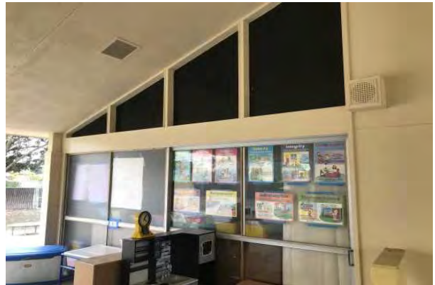
#4 BUILDING 4 - SLIDING DOORS
