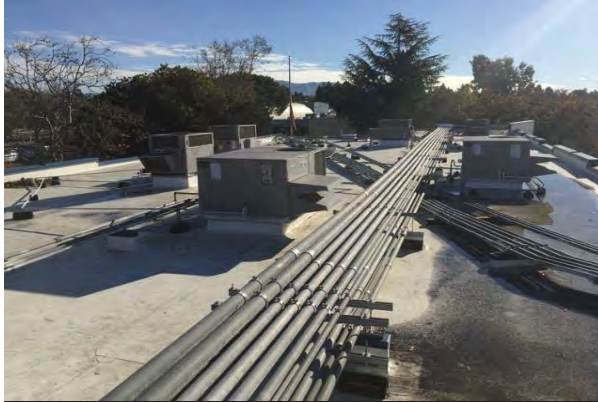
#49 ROOF TOP HVAC UNITS
