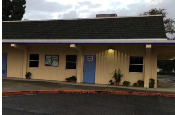
#14 EXTERIOR DOOR AND WINDOW
