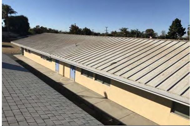
#20 METAL ROOF AT MODULAR BUILDING
