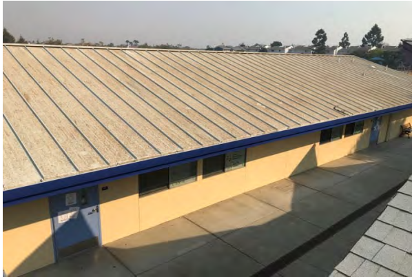
#19 METAL ROOF AT 3A AND 3B
