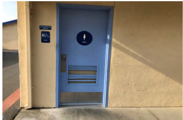
#30 EXTERIOR DOOR AT RESTROOM MODULAR
