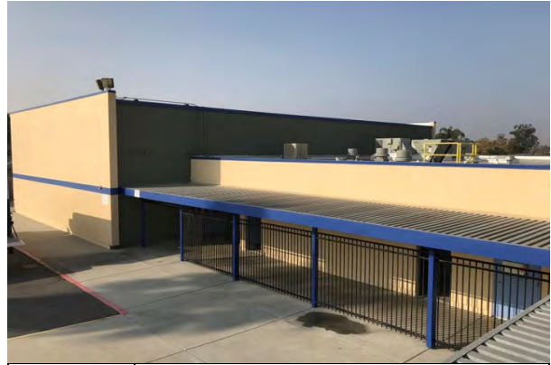
#20 STUCCO WALLS AT MULTIPURPOSE BUILDING
