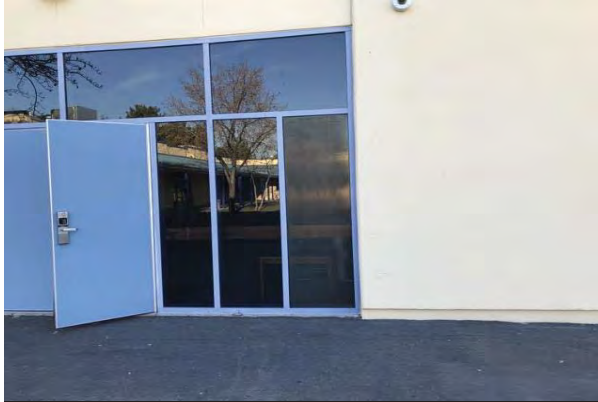
#43 STEEL WINDOWS WITH FIBERGLASS DOORS
