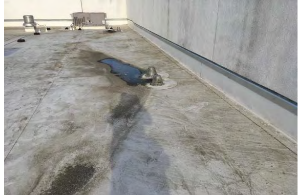
#34 ROOF, SINGLE-PLY TPO
