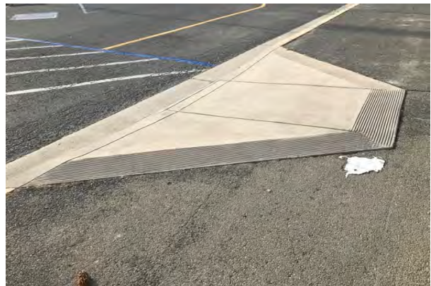
#10 ACCESSIBLE CURB CUT
