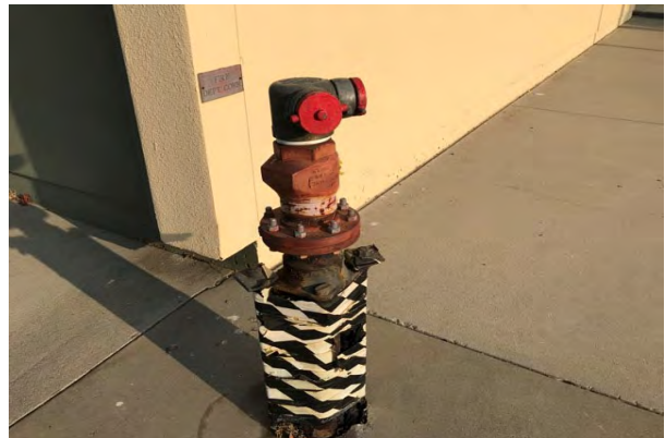
#18 SIAMESE CONNECTOR FOR FIRE SERVICE
