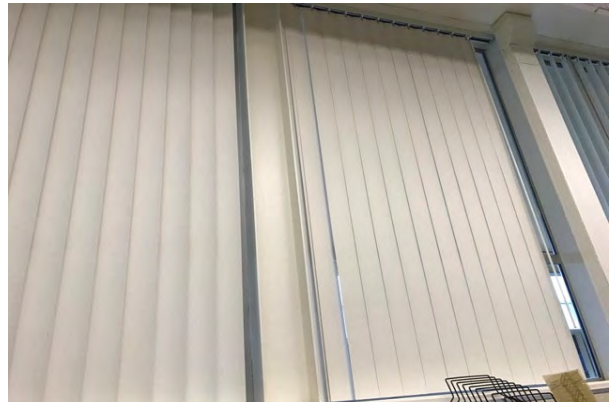
#18 STRUCTURE, STEEL COLUMNS
