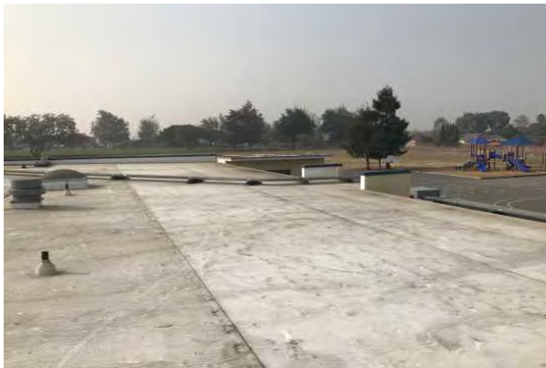
#11 ROOF, TPO MEMBRANE
