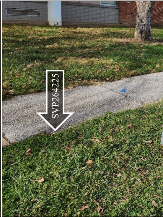
Image 8. Pavement Sediment Southwest of Basketball Courts
