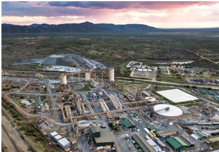
Pilansberg Platinum Mine
