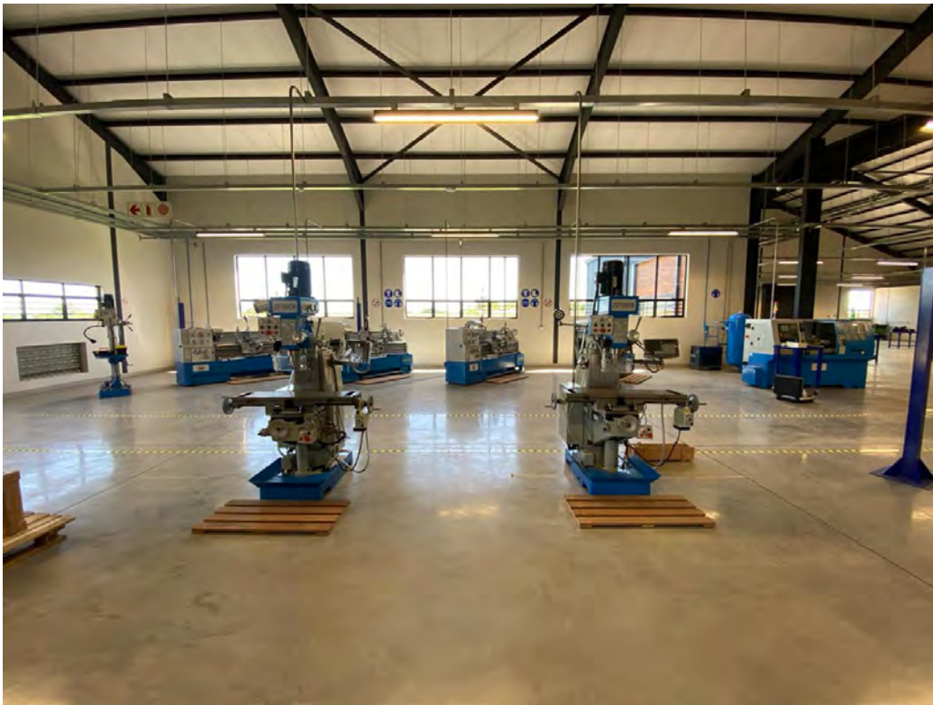
KYB Academy has taken new steps in 2024 to further succeed in technical artisan training by launching its technical training facility in Potchefstroom. TH Machine Tools has supplied conventional lathes and mills
