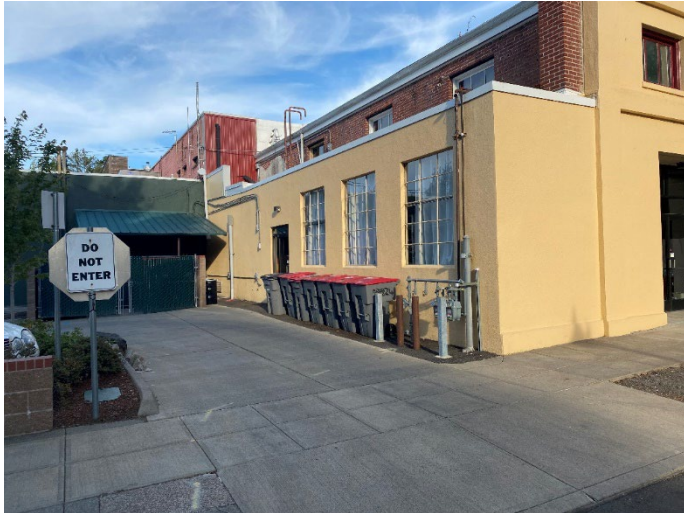
Existing Ford Street Access Location
