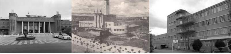
Figures 5, 6, 7. Ankara Railway Station, Ankara Exhibition House, Ankara Girls' High School, respectively [27, 28, 29].
