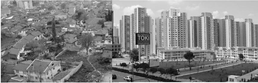
Figure 3. The Project Site Before and After Construction.
