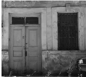
Figure 10. Jamb and Keystone [4].
