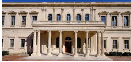
Figure 5. The Entrance Section of Taşkıışla Building Constructed in Neoclassical Style [11].
