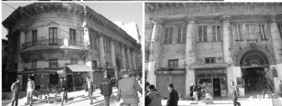
Figure 7. Conditions of the Selected Buildings in 2005 (Karabetça, 2005).
