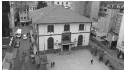
Figure 9. The Rize Orta Mosque before Relocation [17].
