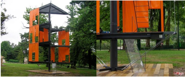
Figure 11. Fiberglass Panels and Iron Used in the Structure of “Deep Purple” by Massimiliano and Doriana Fuksas.
