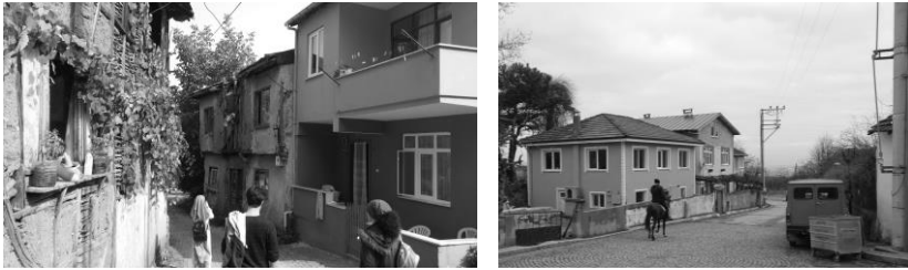
Figure 23. Reinforced Concrete Structures in the Village (Uzuner Archive, 2015).
