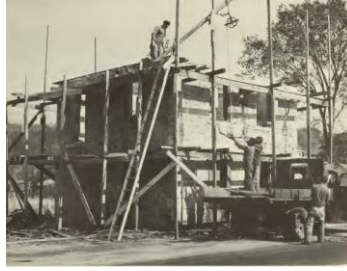
Figure 2. Disassembly of the Mystic Bank [7].
