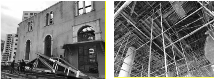
Figure 17. Wood Ceilings and Beams.
