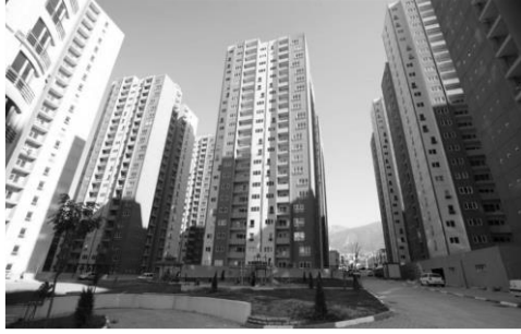
Figure 4. An Inner View from Doğanbey Urban Renewal Project.
