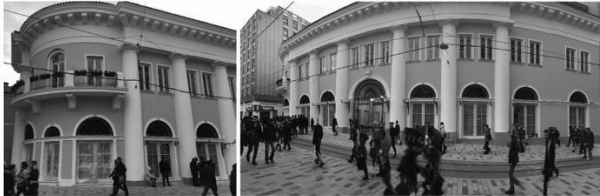
Figure 8. Current Conditions of the Selected Buildings in 2019 (Karabetça, 2019).
