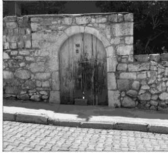
Figure 7. A Courtyard Gate in Kale Constructed with the Replaced Building Material, 2019.
