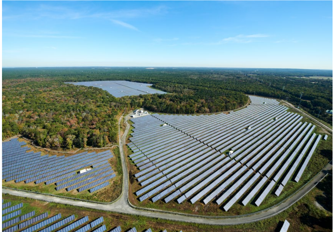
32 Megawatt Long Island Solar Farm, Upton, New York
