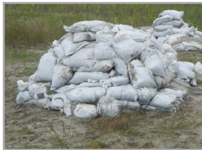
Sand Bag Mitigation Completed Prior to Intentional Detonation
