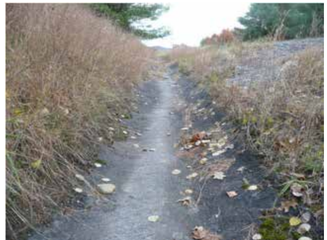
Close-up Photograph showing Asphalt Swales along I-87.
