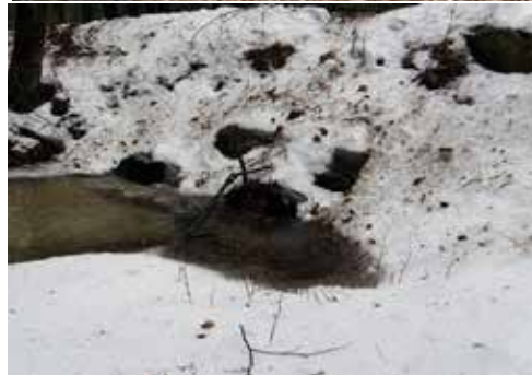
The two pipes are not working in this application/site. During storm events this culvert clogs up, backs up water, which then washes out the road. This is a problem area that causes crews to attend to it every time Westport gets a large storm. Photos of the inlet also depict an unstable slope due to past washouts.
