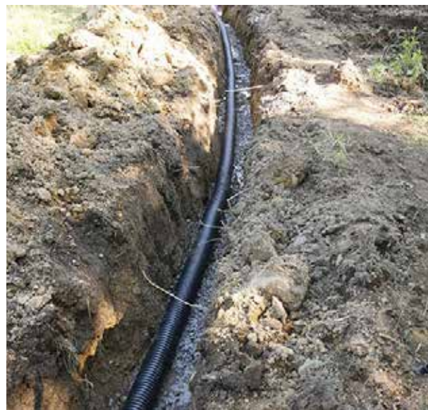
Image of tile ditch with perforated corrugated pipe for drainage (tile drain). Photo credit: Deerbuilder.com
