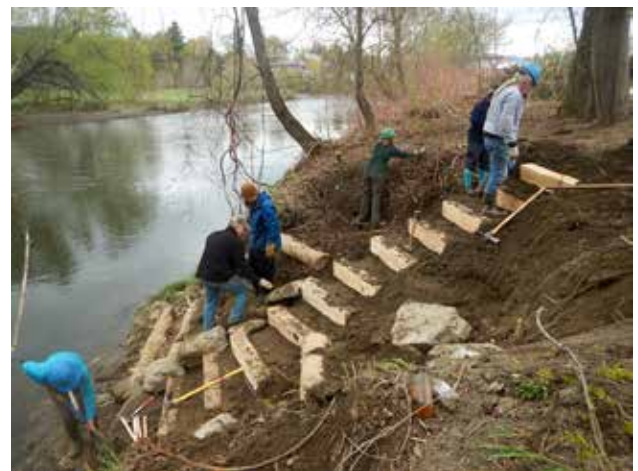
Volunteers stabilizing an eroding bank along the Lamoille River. Spring 2017
