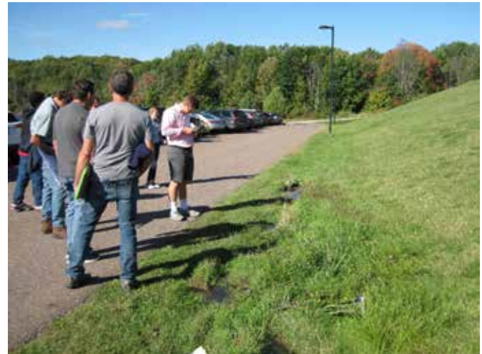
CVU students study the eroding swale north of the parking lot.
