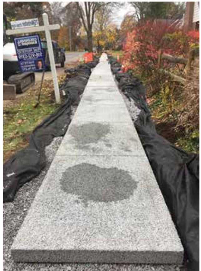
Pervious concrete sidewalk section installed in Glens Falls in 2018
