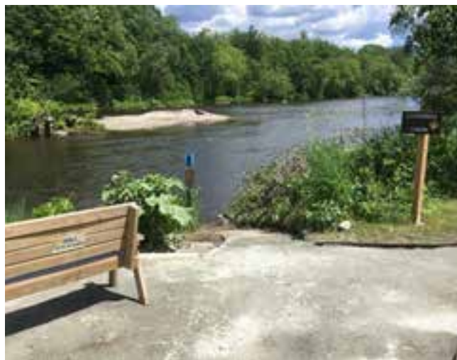
Completed accessible trail, ramp, and bench
