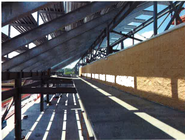
J. Fred Johnson Stadium –Lower Level Press Box Framing.
