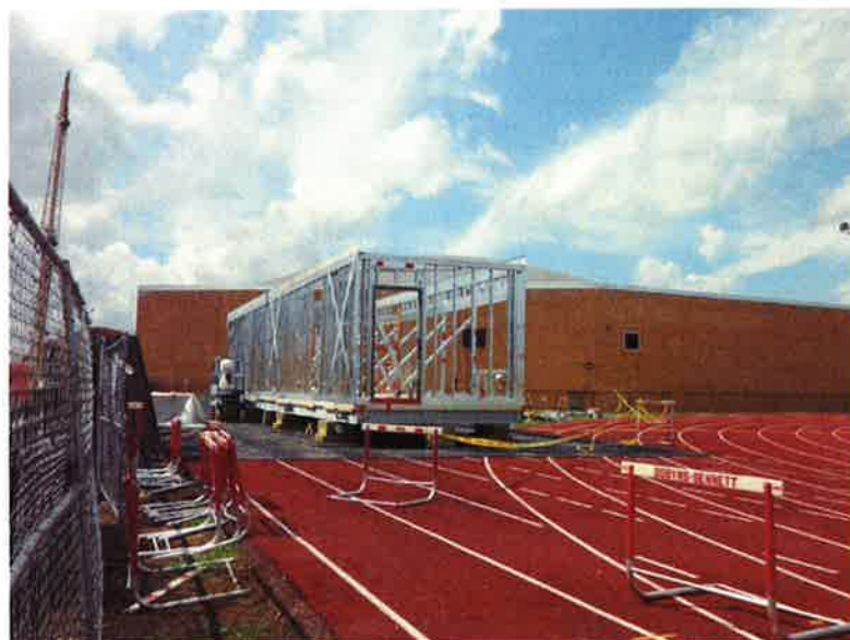
J. Fred Johnson Stadium –Lower Level Press Box Framing.
