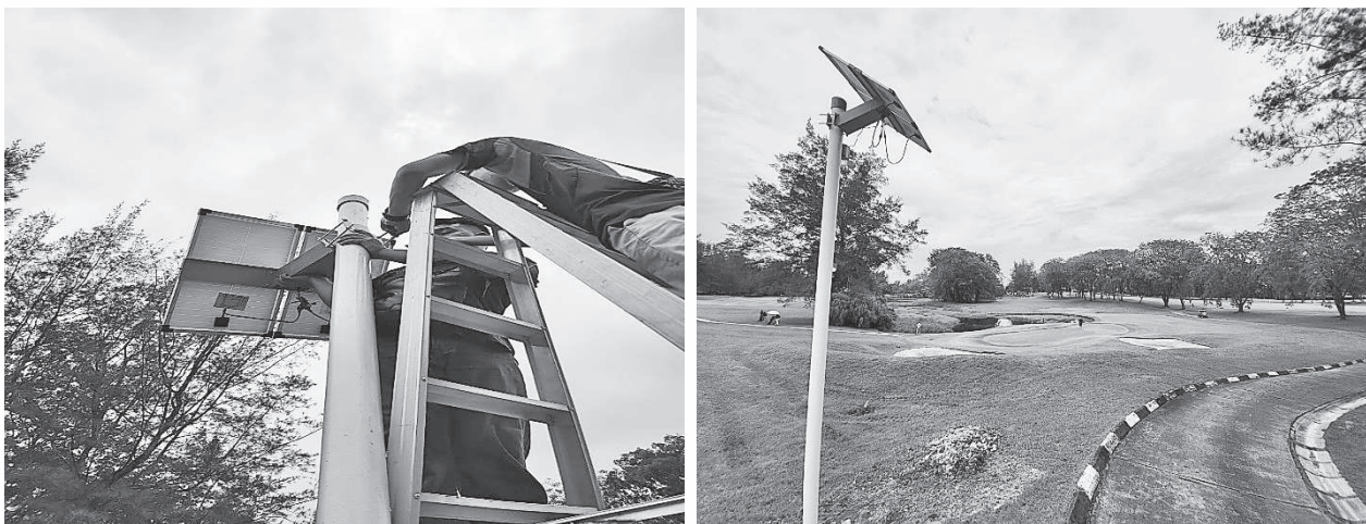
Installation completion at Matang Hole 3 on 21 st October 2022
