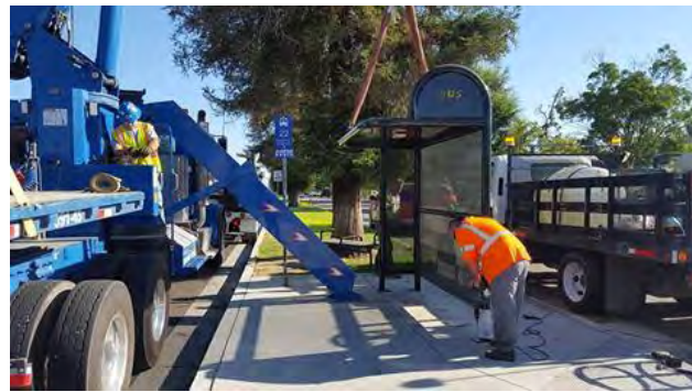
Installation of new bus stop
