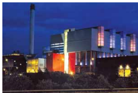
Tysley Waste-to-Energy plant, Birmingham, UK. Built in 1996, the 28 MW plant with a 2-stream incinerator has a combined capacity of over 350,000 tonnes per year of municipal solid waste and a fifteen year Non-Fossil Fuel Obligation Contract. An award winning lighting system illuminates the plant at night.
