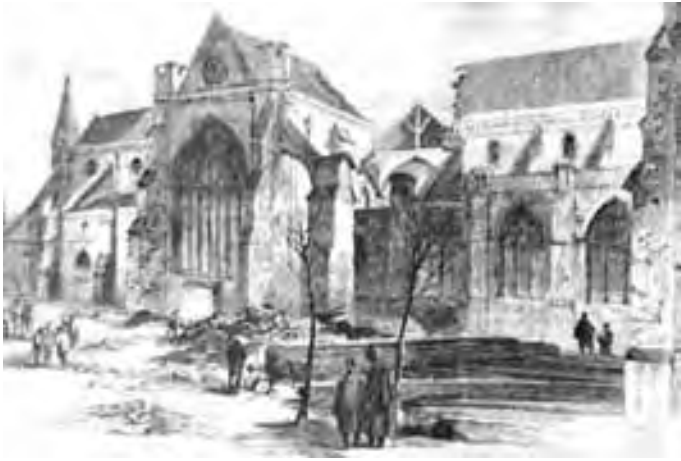
Figure 275. Chichester Cathedral after collapse of the central tower in 1861
