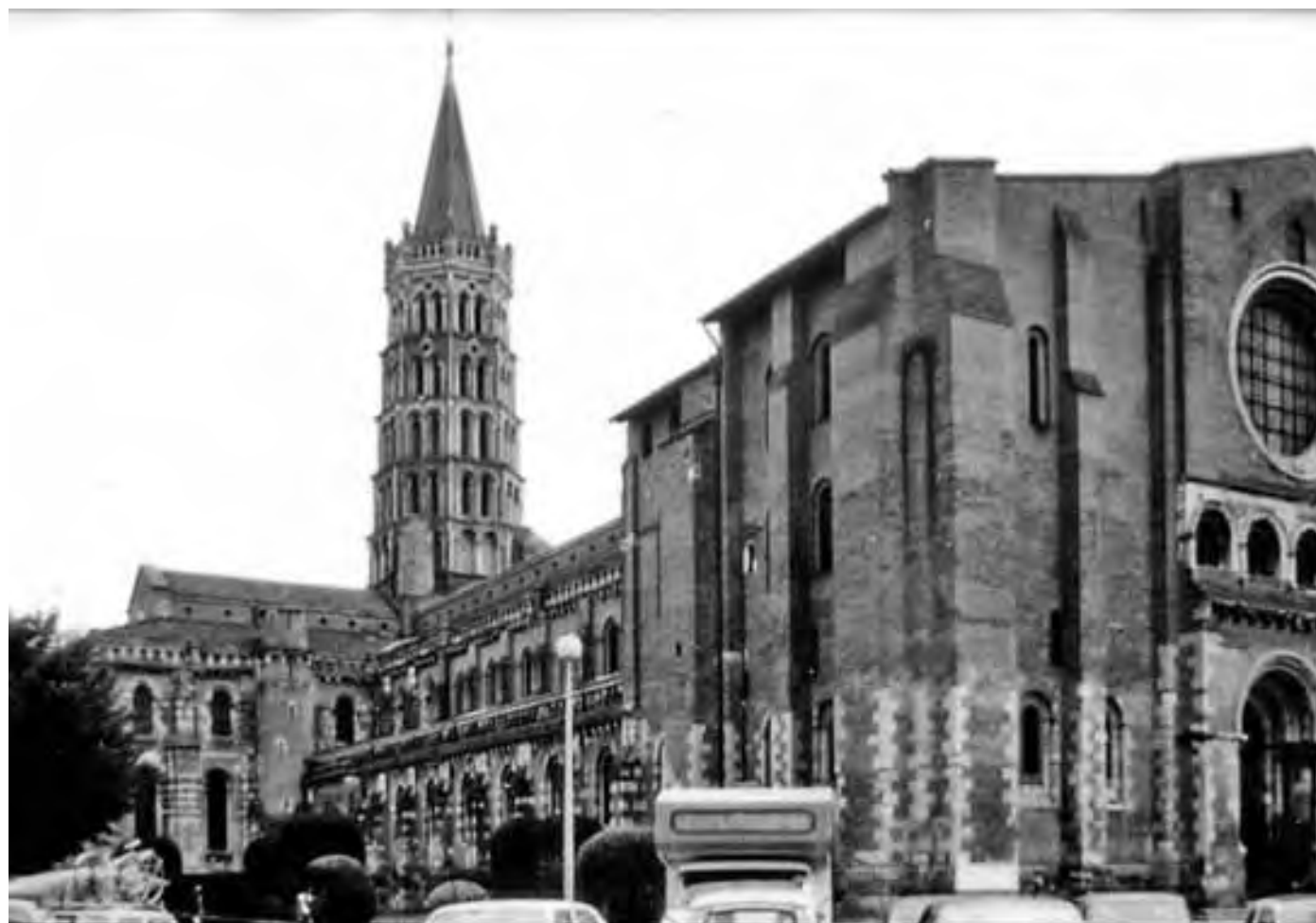
Figure 257 (below). Toulouse, Saint-Sernin, north elevation after Viollet-le-Duc's restoration. The building was transformed from Romanesque to Gothic (photo 1980)
