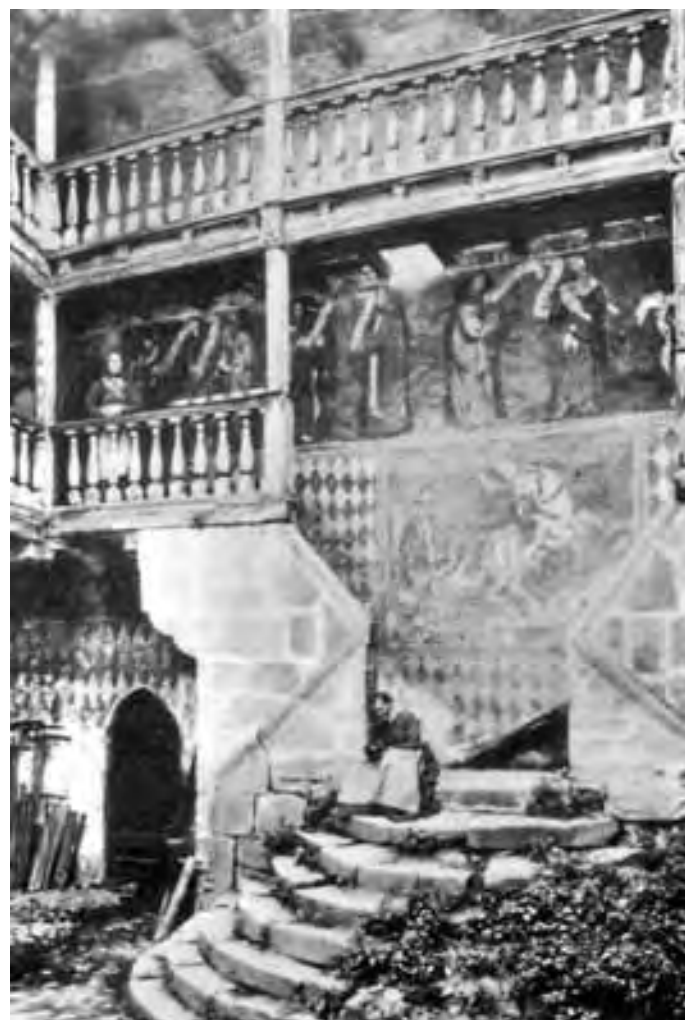
Figure 302. Castle of Fénis, Piedmont: courtyard before restoration (prior 1897). This castle served as a model for the 'Borgo' in 1884
