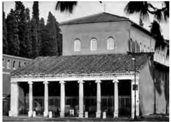
Figure 338. San Lorenzo fuori le mura, Rome, rebuilt after damages in the Second World War
