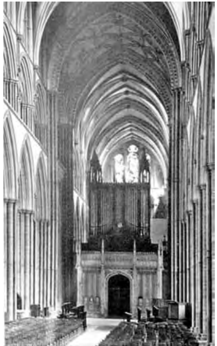
Figure 211. Salisbury Cathedral, c. 1865, showing screen designed by Wyatt
