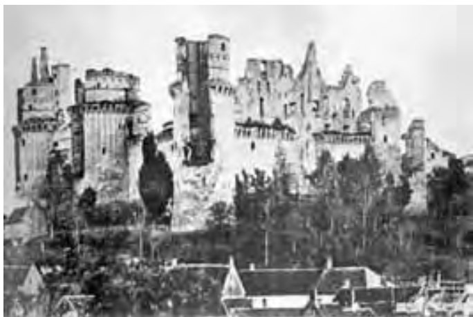
Figure 262. The Castle of Pierrefonds before restoration
