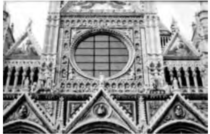
Figure 296. Siena Cathedral, west front after restoration
