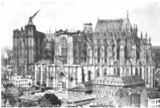
Figure 232. Cologne Cathedral with its surroundings during the construction, 1855 (photo J.F. Michiels)
