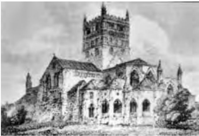
Figure 290. Tewksbury Abbey before restoration. Its proposed restoration by Scott caused William Morris to write a letter in the Athenaeum and call a meeting for the foundation of SPAB
