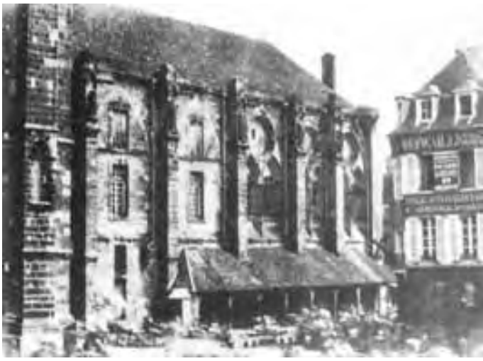
Figure 258. Sens, Bishop's Palace before restoration (photo 1851)
