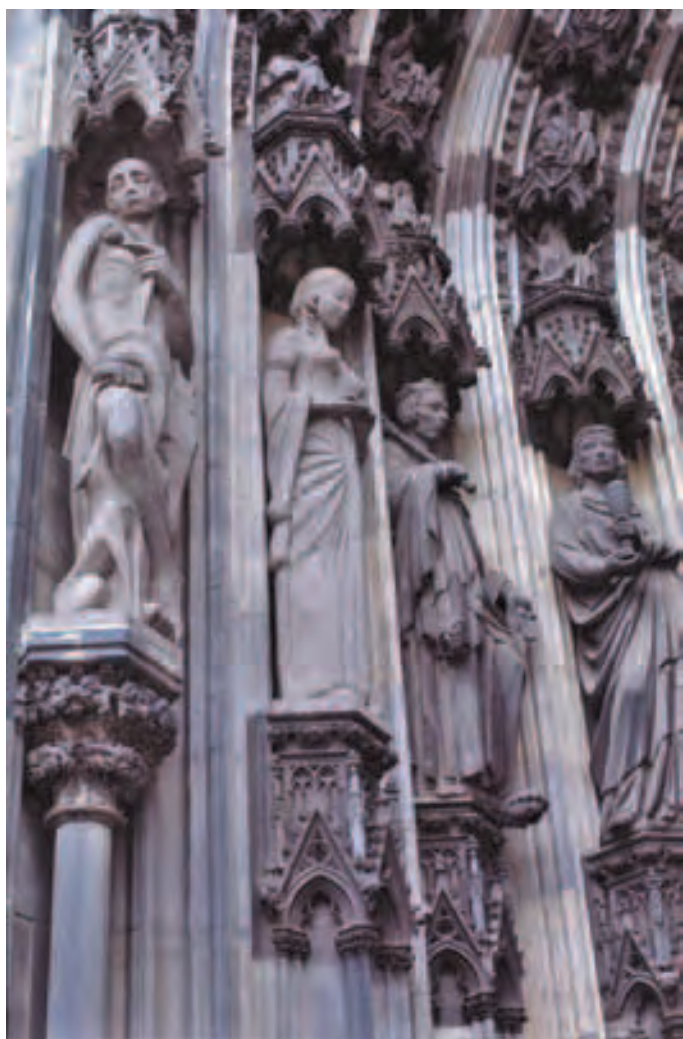
Figure 233. Cologne Cathedral, south transept entrance including also modern statues from restoration after the Second World War
