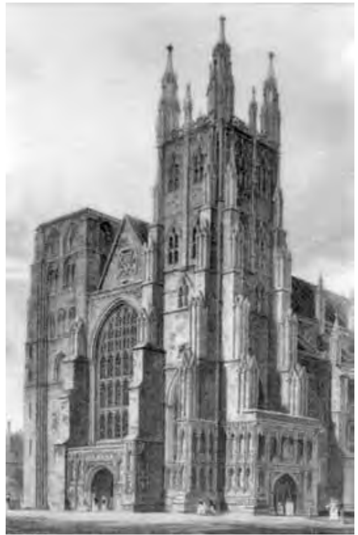
Figure 269. Canterbury Cathedral before restoration
