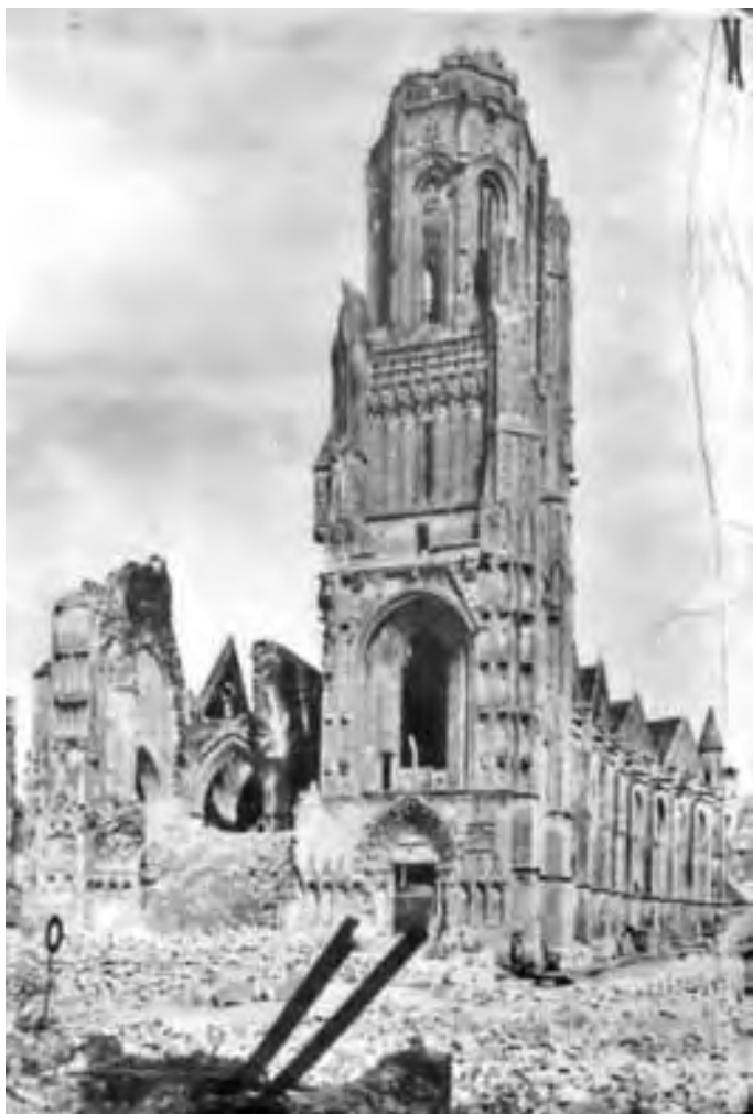
Figure 238. Notre-Dame of Saint-Lô destroyed in the Second World War
