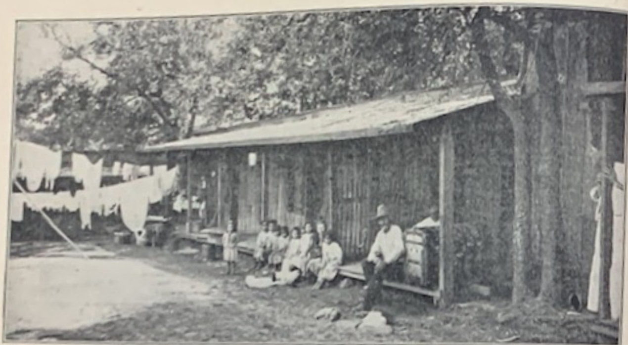
THE WORST SECTION OF THE CONTINUOUS CORRAL.
