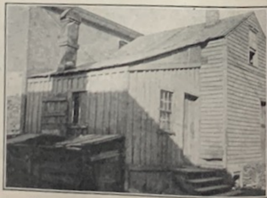
MANURE BOX UNDER A KITCHEN WINDOW.
