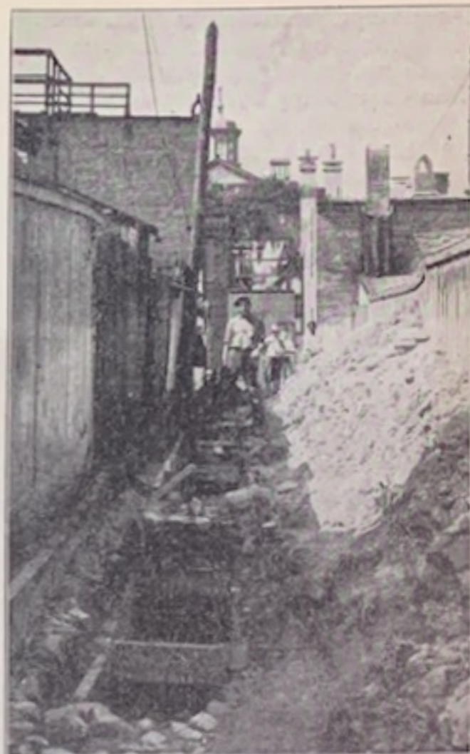
SEWER IN AN ALLEY.
