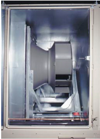
Figure 4: SWSI airfoil plenum fans
