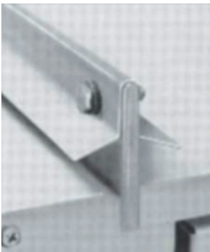
Figure 1: Standing top seam
