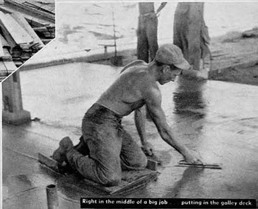
The mess hall again. Should be ready by supper-time.
