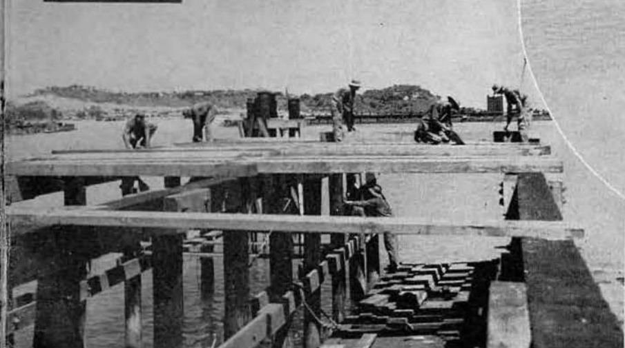
Putting in the deck.
