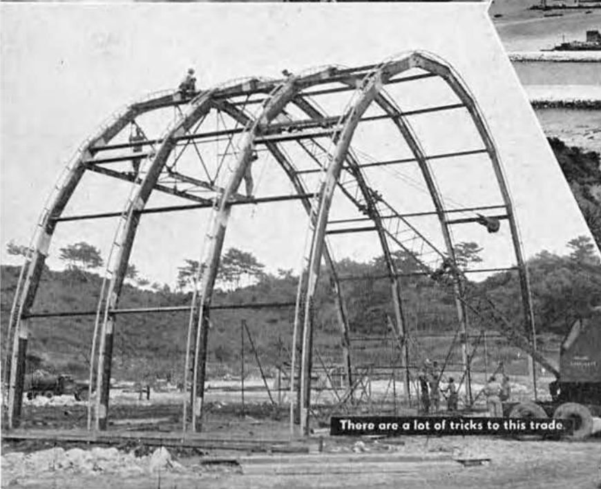
Beams and ribs are bolted into place.
