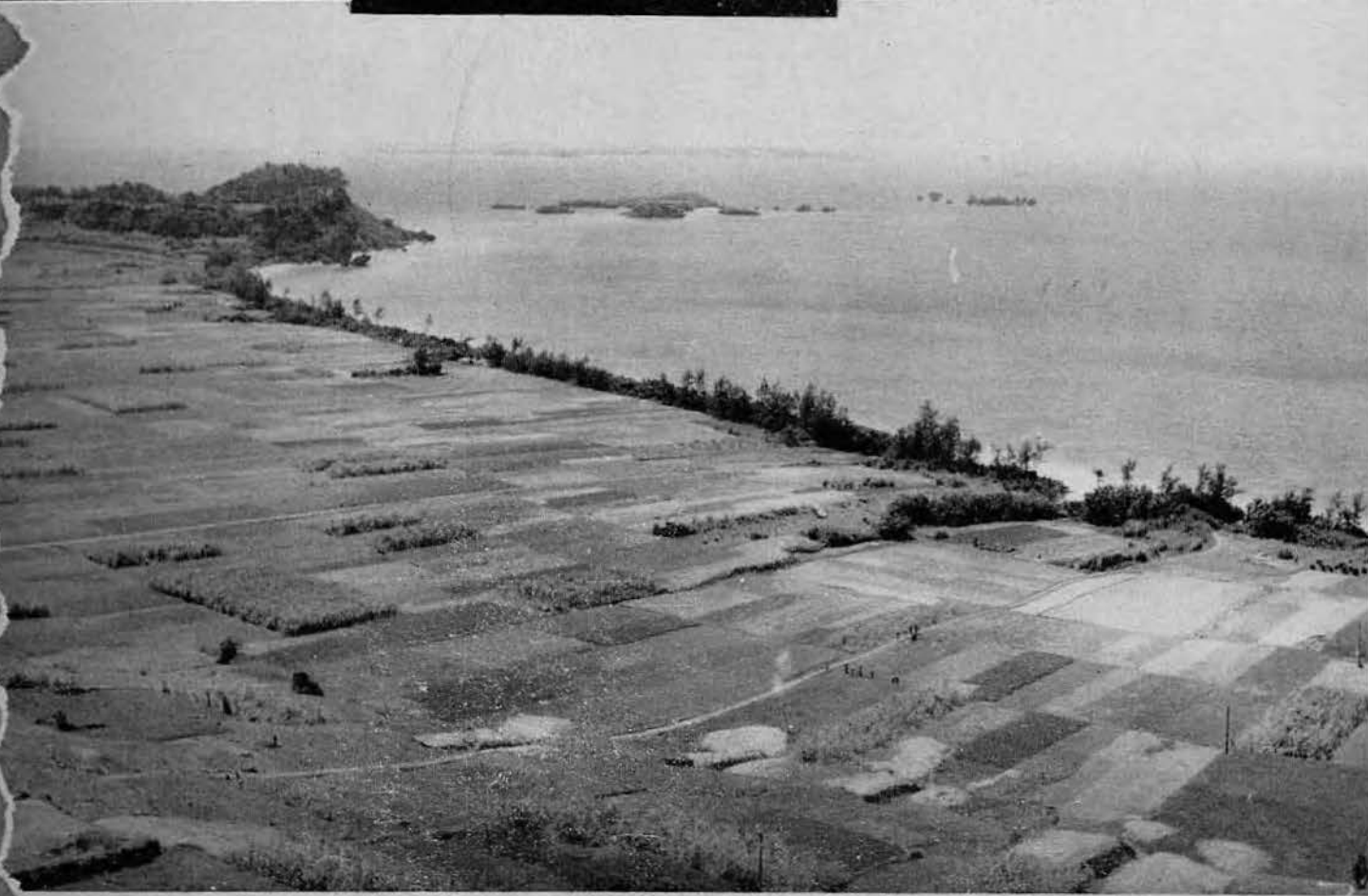
It looked like this before we started.
