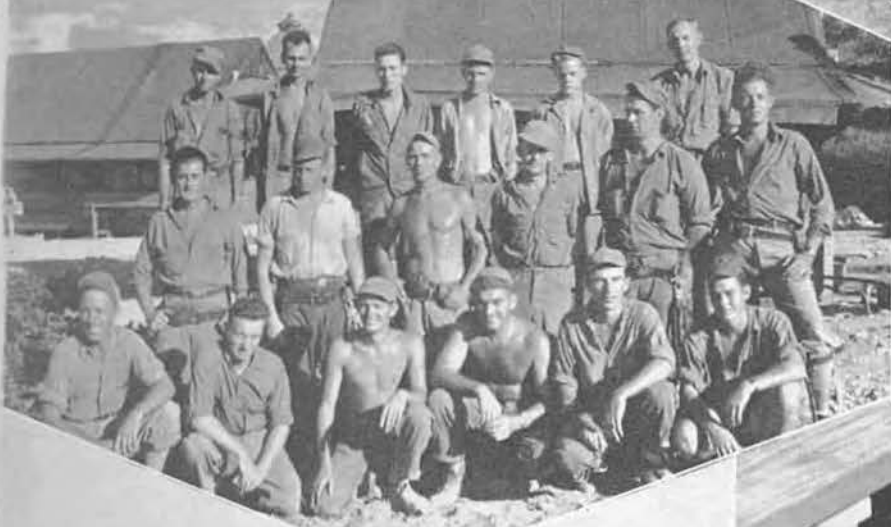
Electrical and Telephone gang
