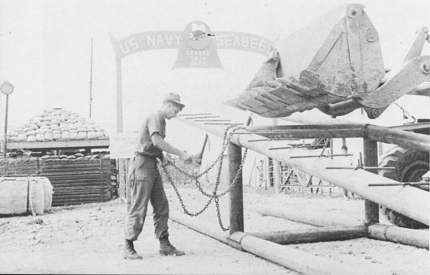
EO3 James Crusan of 0604 prepares a steel tower for placement.
