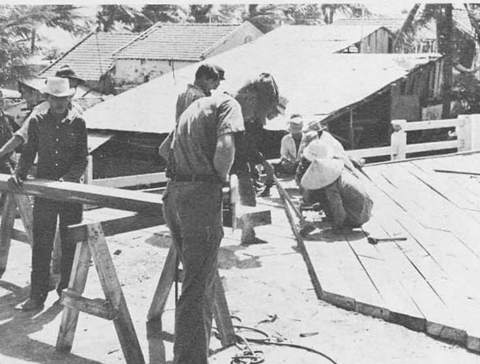
0603 builds a bridge in Phang Rang City.
