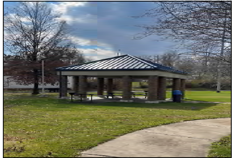
4) View of onsite picnic shelter.
