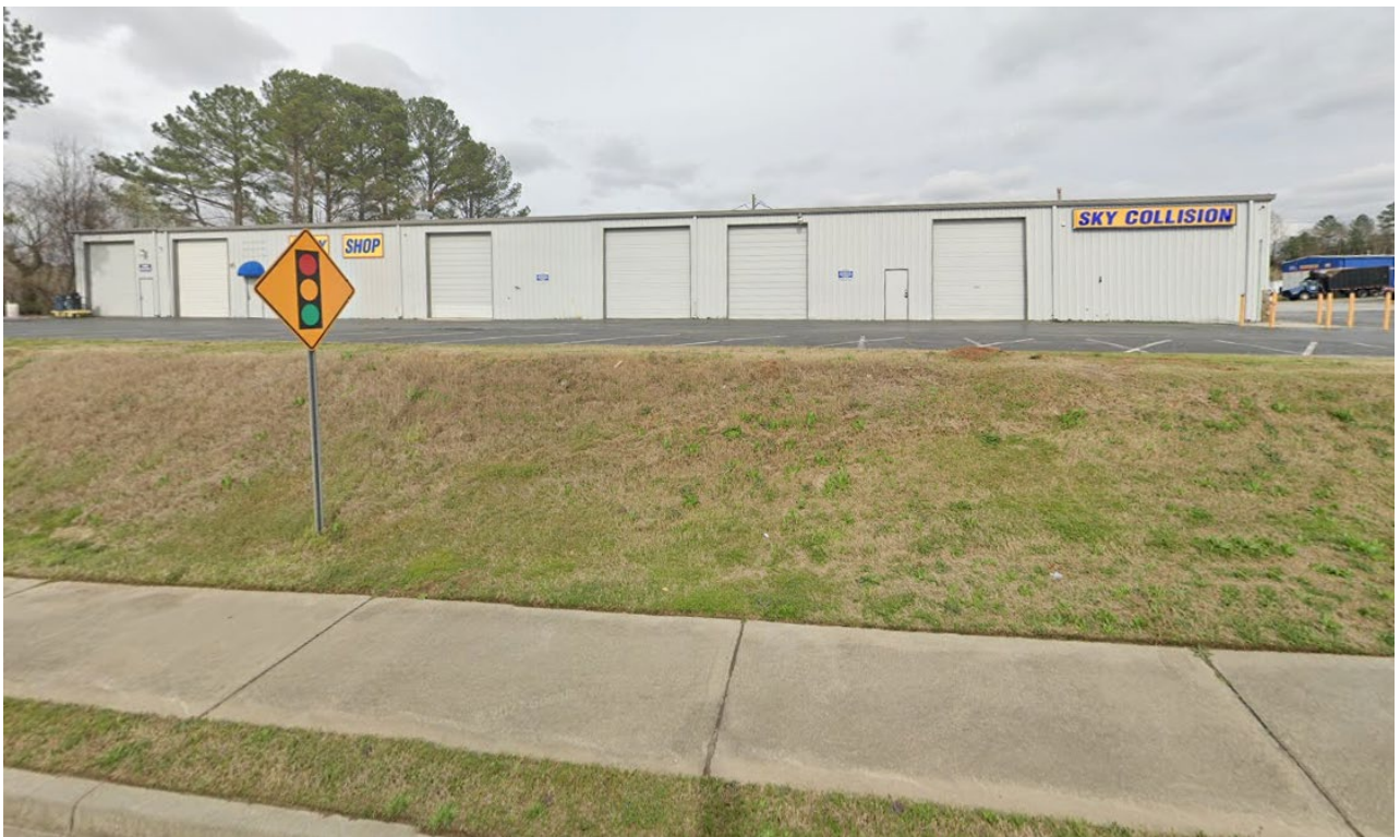
Bays on west side of building along Arcado Road
