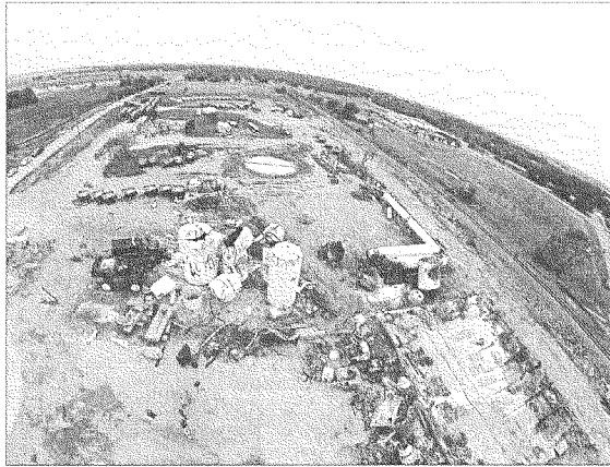
Figure 1: Photographs of Damage from the Explosion in West, Texas in April 2013
