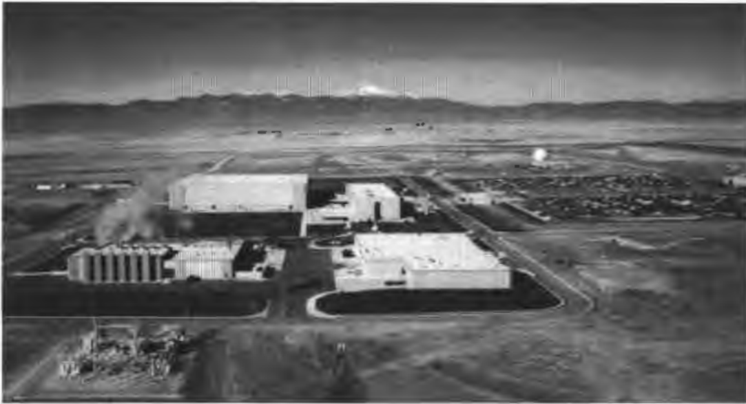
Illustration 9-1 Schriever AFB and the Jack Swigert Space Operations Facility – the large building at the top left
