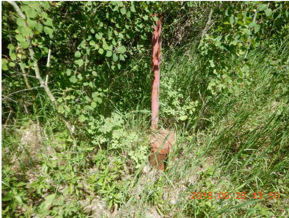
Photo 13 - Well MW13 – Casing Locked
