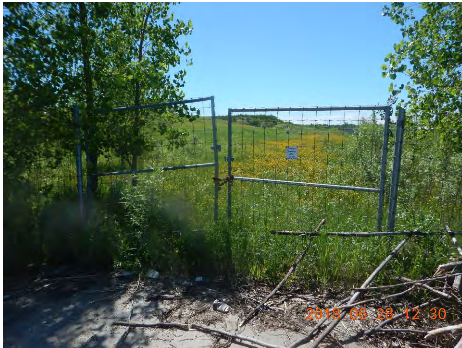
Photo 32 – Containment Cell Area Entrance Gate – Locked at Completion of Cell Inspection
