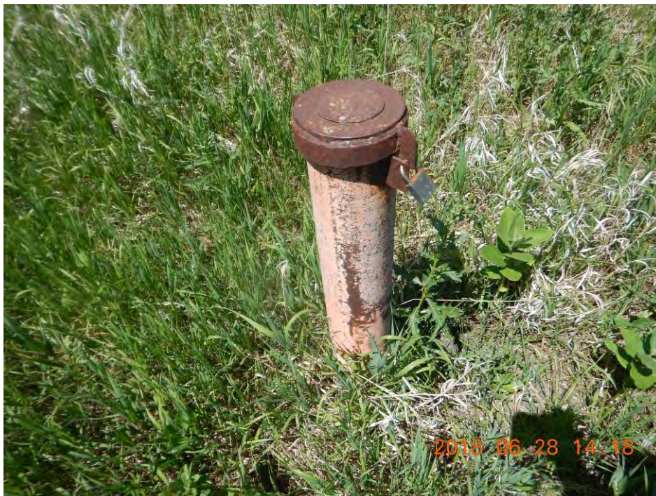
Photo 14 - Well MW14 – Casing Locked and Welded
