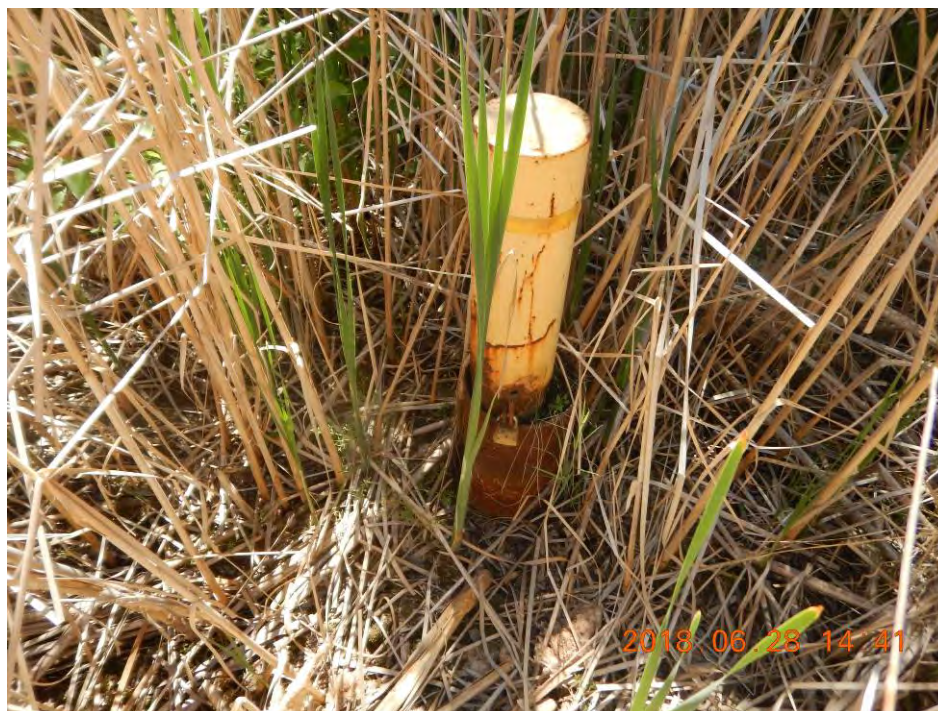
Photo 18 - Well 2000-B4 – Casing Locked and Welded
