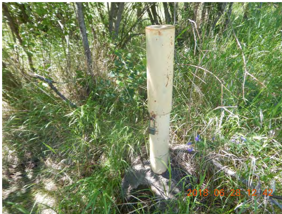
Photo 25 - Well 99-Cell-1 – Casing Locked
