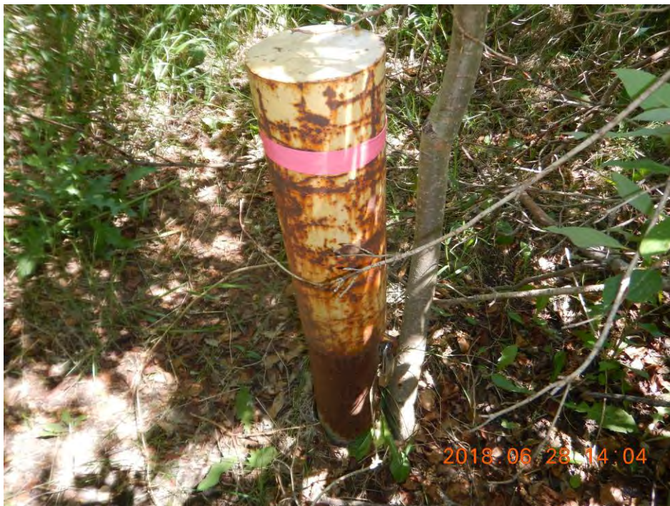
Photo 4 – Well MW3 – Casing Locked
