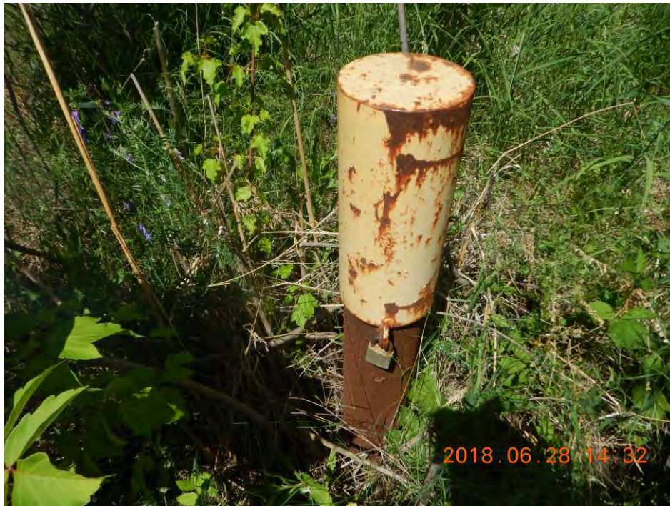
Photo 16 - Well 2000-B2 – Casing Locked
