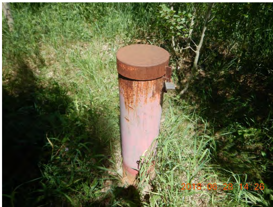
Photo 10 - Well MW10 – Casing Locked
