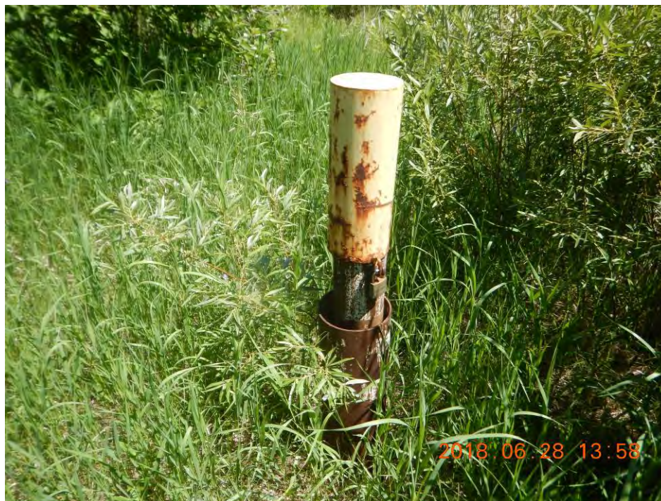
Photo 17 - Well 2000-B3 – Casing Locked and Welded
