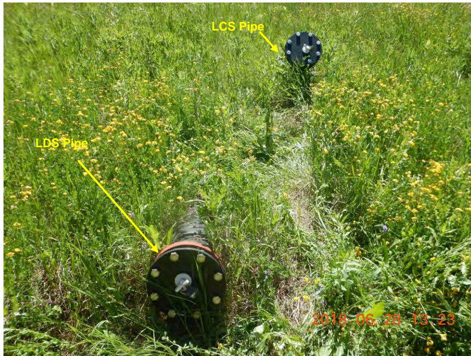
Photo 29 – Leachate Collection and Leakage Detection System (LCS and LDS) Access Pipes North Side – Locked and Secure
