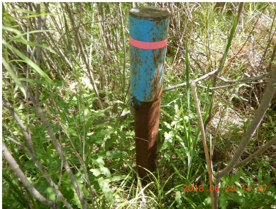
Photo 19 - Well 2002-B5 – Casing Locked and Welded
