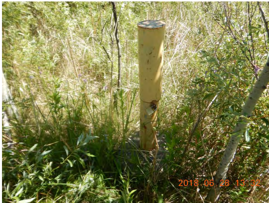
Photo 28 – Well 99-Cell-4 – Casing Locked
