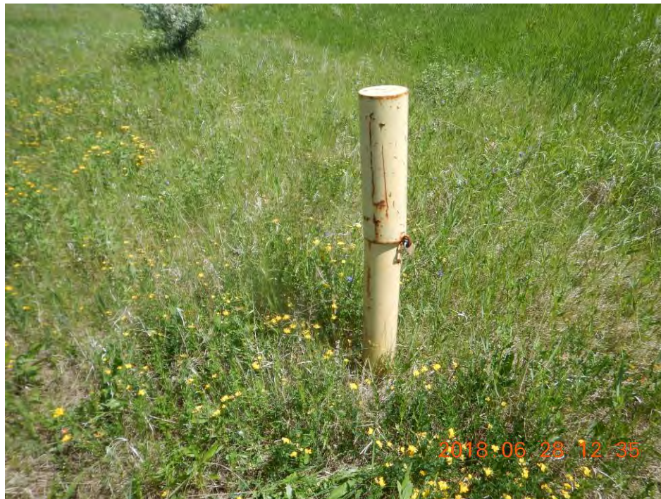
Photo 26 - Well 2003-Cell-2 – Casing Locked
