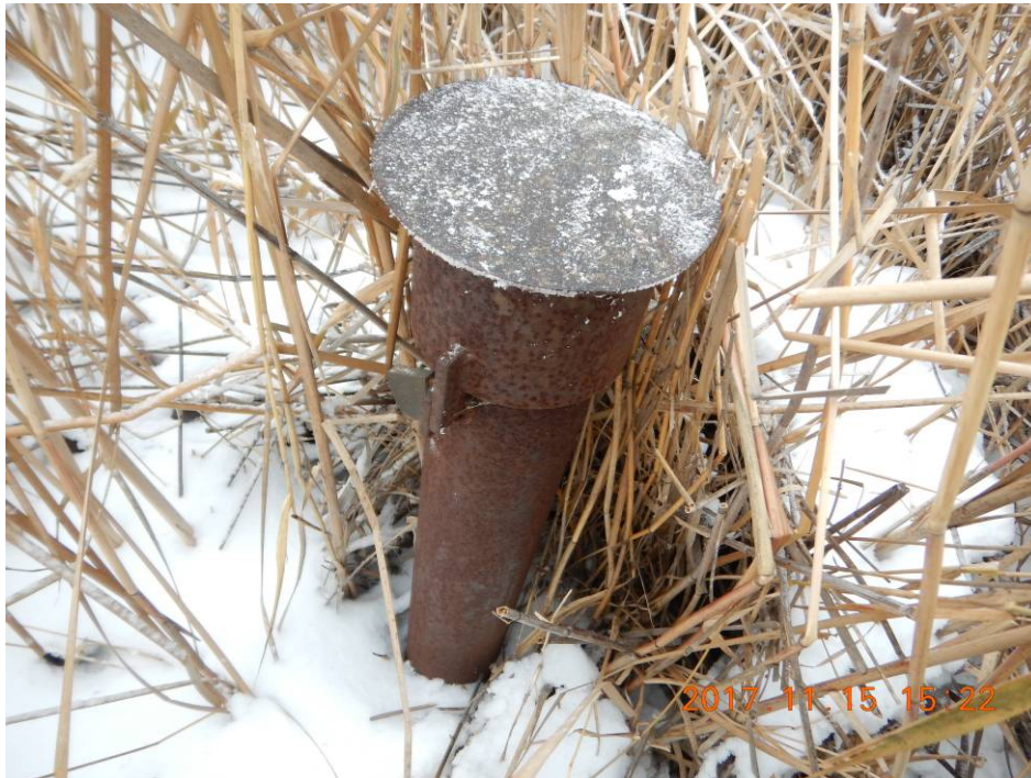
Photo 8 – Well MW8 – Casing Locked and Welded
