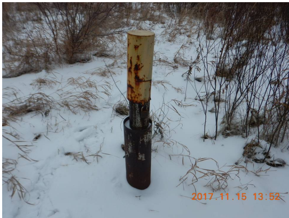
Photo 17 - Well 2000-B3 – Casing Locked and Welded
