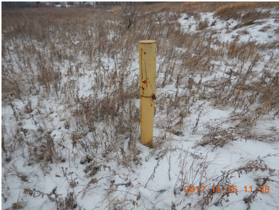
Photo 26 - Well 2003-Cell-2 – Casing Locked
