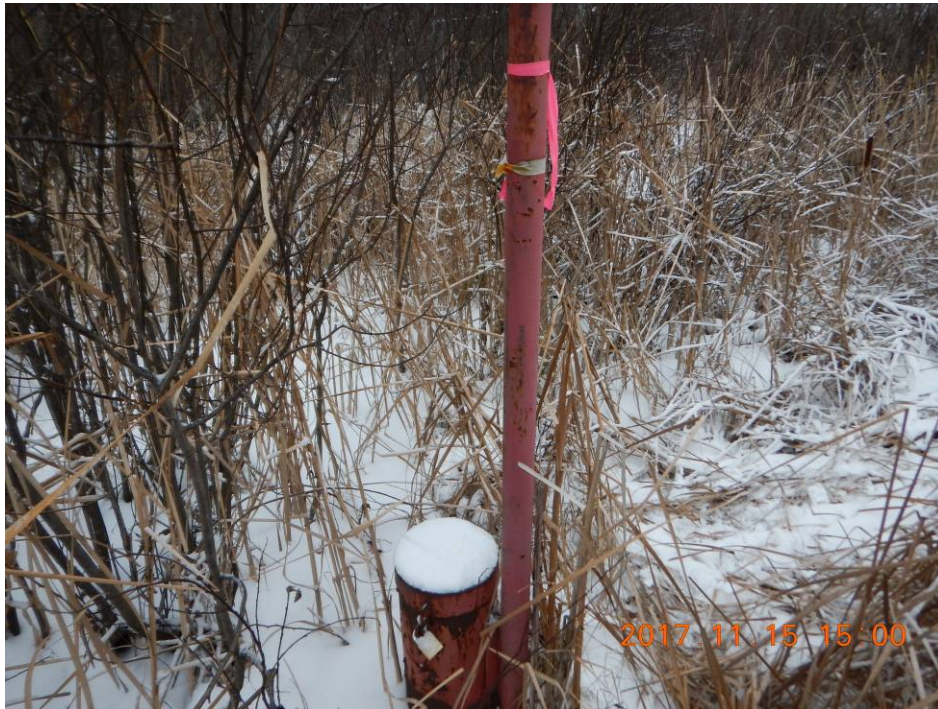
Photo 9 - Well MW9 – Casing Locked and Welded
