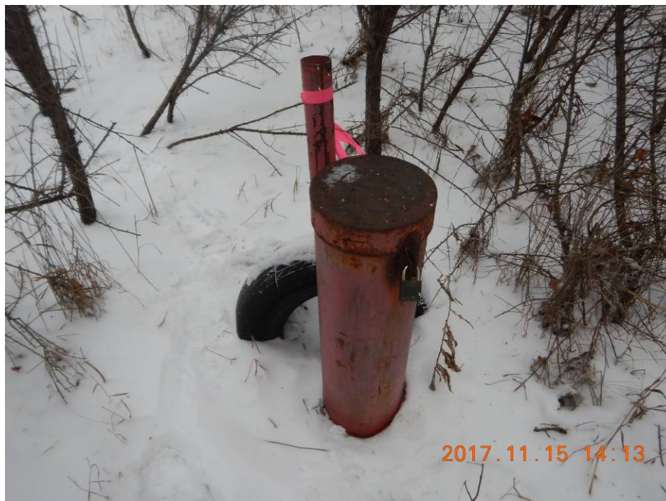
Photo 11 - Well MW11 – Casing Locked
