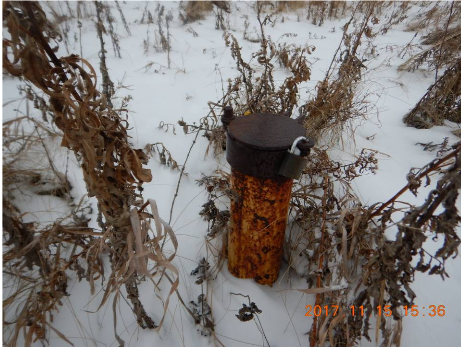
Photo 7 – Well MW7 – Casing Locked and Welded
