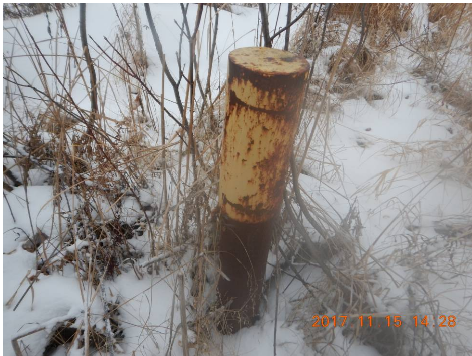
Photo 16 - Well 2000-B2 – Casing Locked
