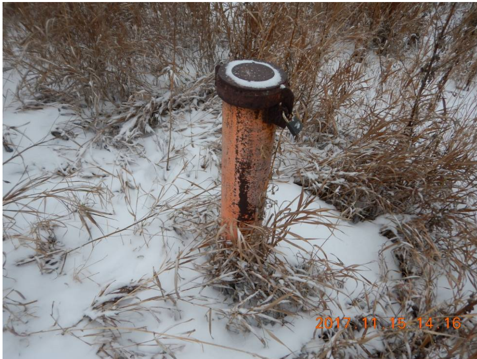
Photo 14 - Well MW14 – Casing Locked and Welded
