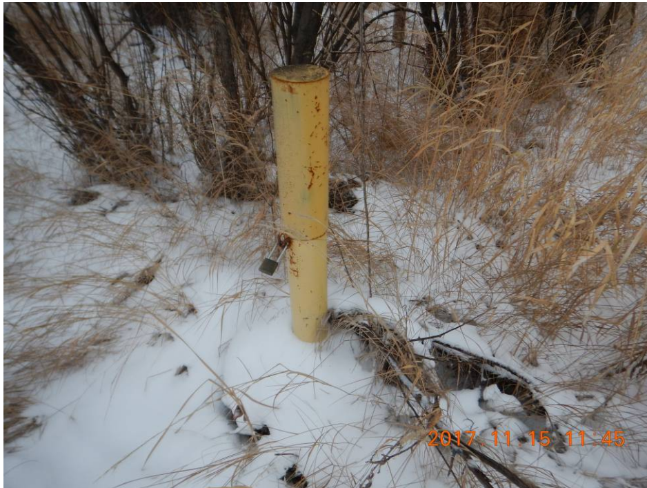
Photo 25 - Well 99-Cell-1 – Casing Locked
