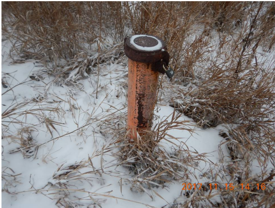
Photo 10 - Well MW10 – Casing Locked
