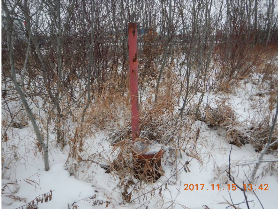
Photo 13 - Well MW13 – Casing Locked
