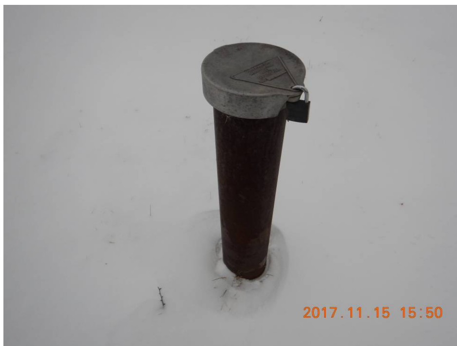
Photo 20 - Well 99-B1 – Casing Locked
