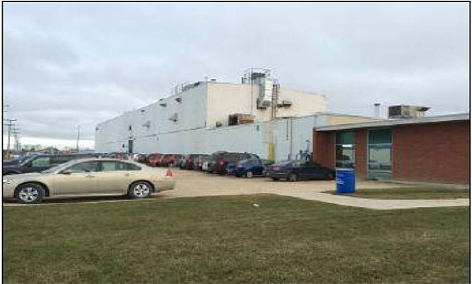
View of west side of Site building.
