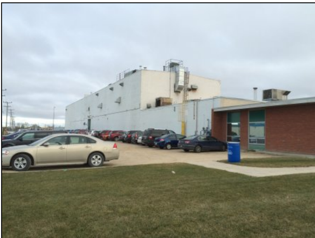
View of west side of Site building.
