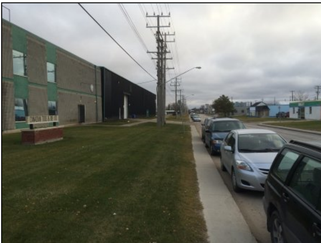
View of south side of Site building looking east.
