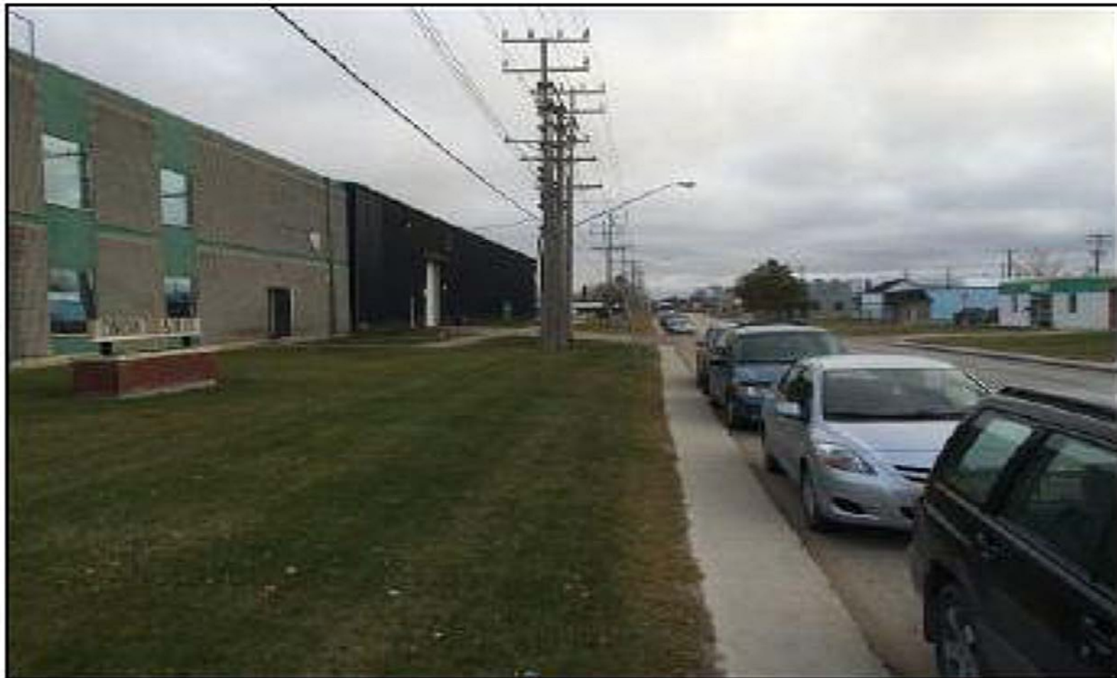
View of south side of Site building looking east.
