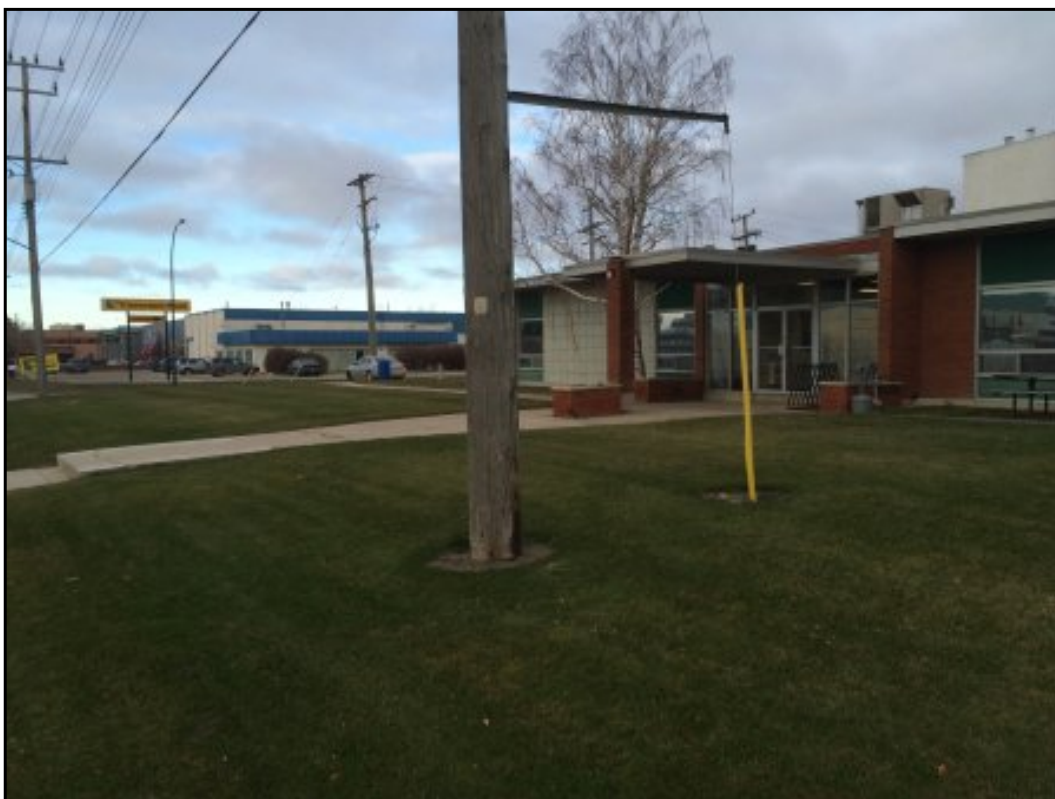
View of southwest corner of Site building, looking west.
