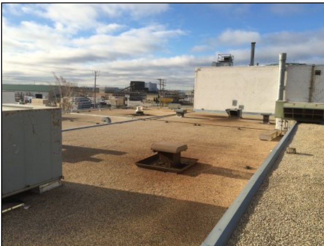
View of Site building rooftop.
