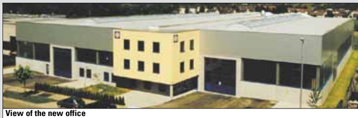
View of the new office
