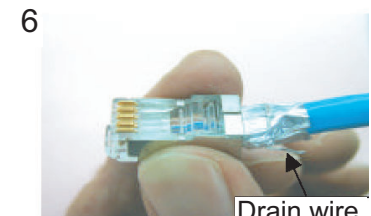
Insert the cable into the modular plug so that the folded part of the shield enters into the plug housing. The drain wire should be located on the tab side of the jack.
