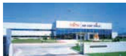
Fujitsu General (Thailand) Co., Ltd. (Thailand)
