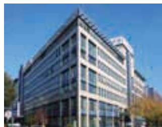
R&D Center in Fujitsu General (EURO) GmbH (Germany)
