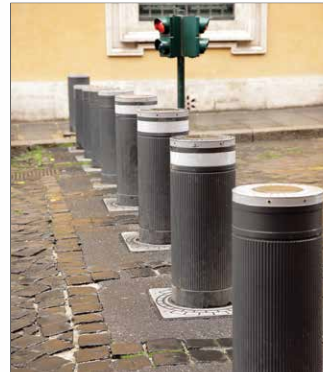
In this road barrier application, the linear motion is provided by an inverted keyed machine screw jack.
