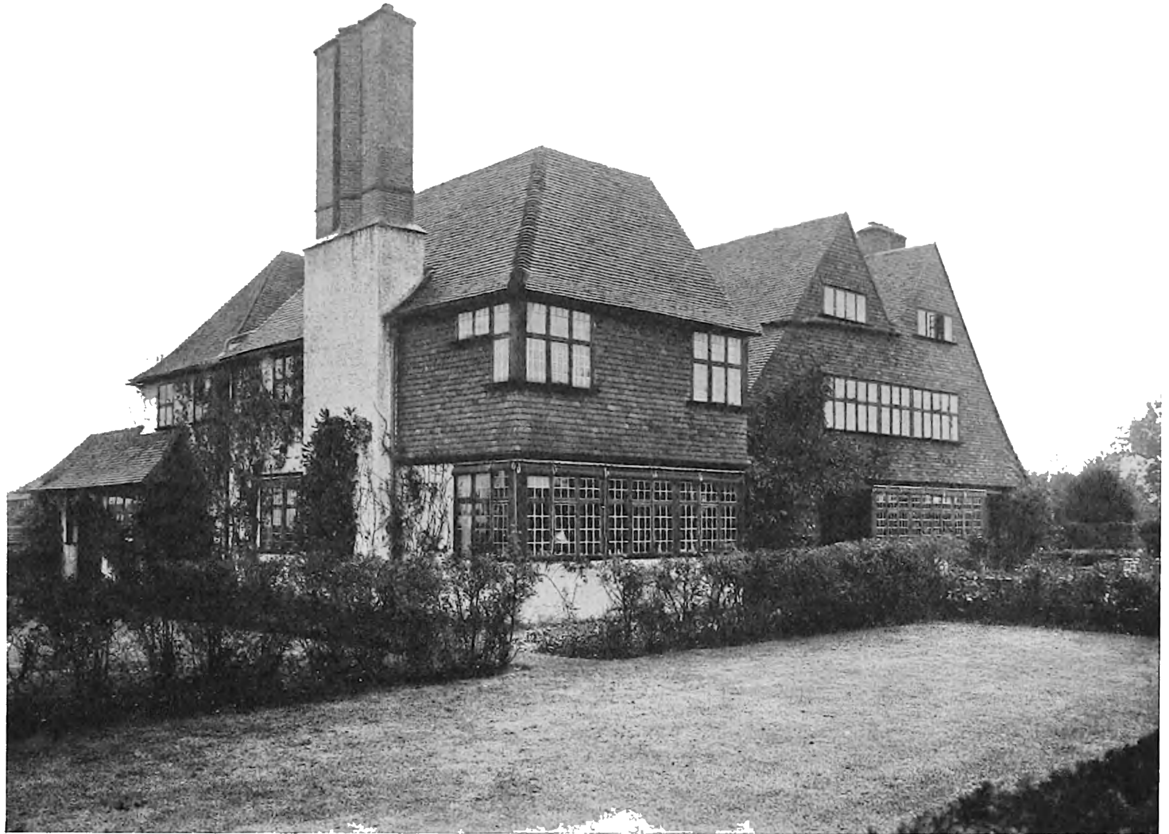
BERRYDOWN COURT, OVERTON : SOUTH FRONT
