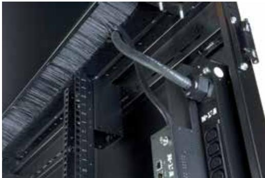
RP Series rack with 2 installed Eaton ePDUs
